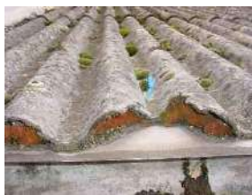
Asbestos cement roof sheeting
