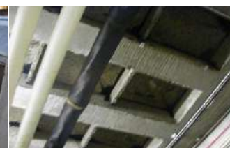
Sprayed ceiling coatings
