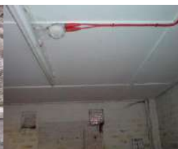
Ceiling asbestos insulating board
