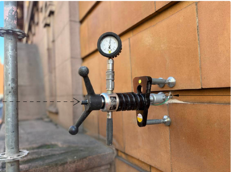
Image 02 - Typical Eyelet/anchor and location within Recesses Rusticated Terracotta
