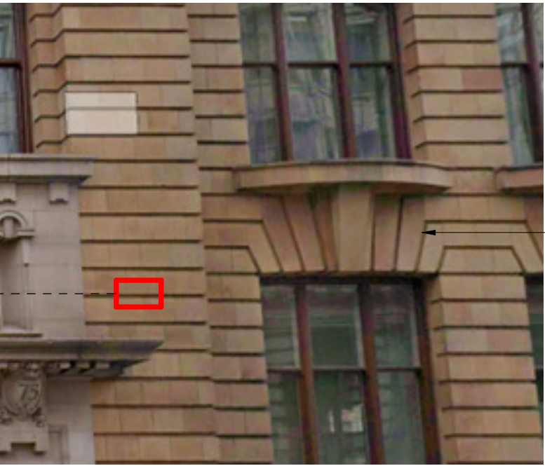
Image 01 - Approximate location of pull test (Red Square)
