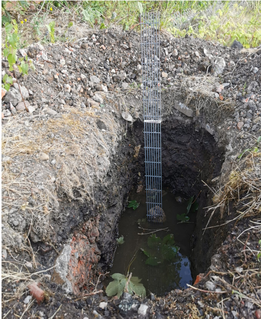
5. Trial pit A with 25% water left
