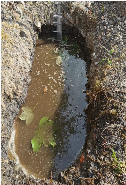
7. Trial pit A with full water
