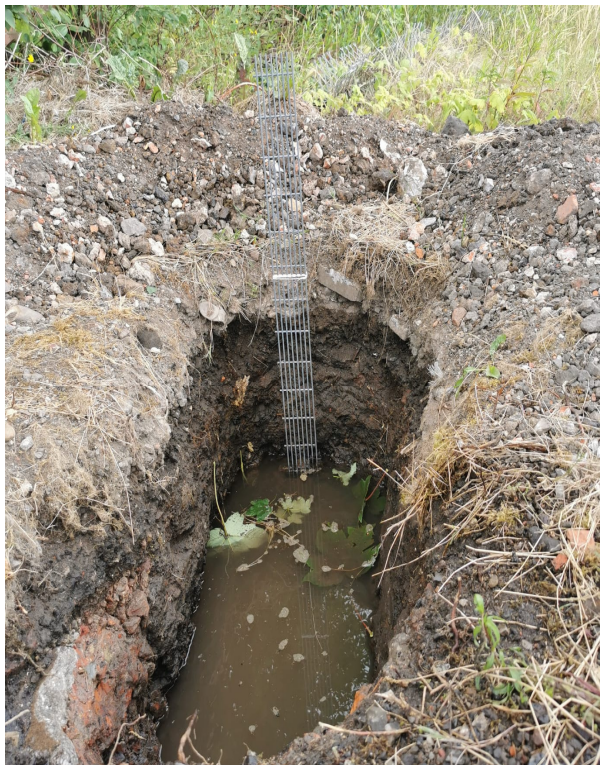
8. Trial pit A -half water
