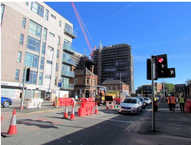
View North-east Along Rochdale Road, Towards Application Site
