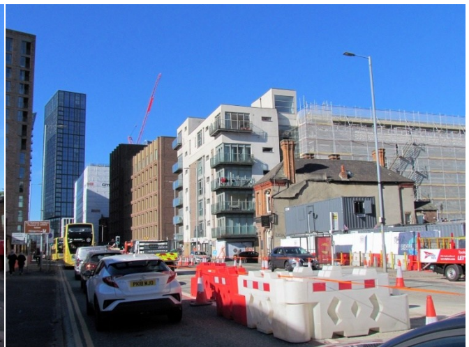
View South-west Along Rochdale Road
