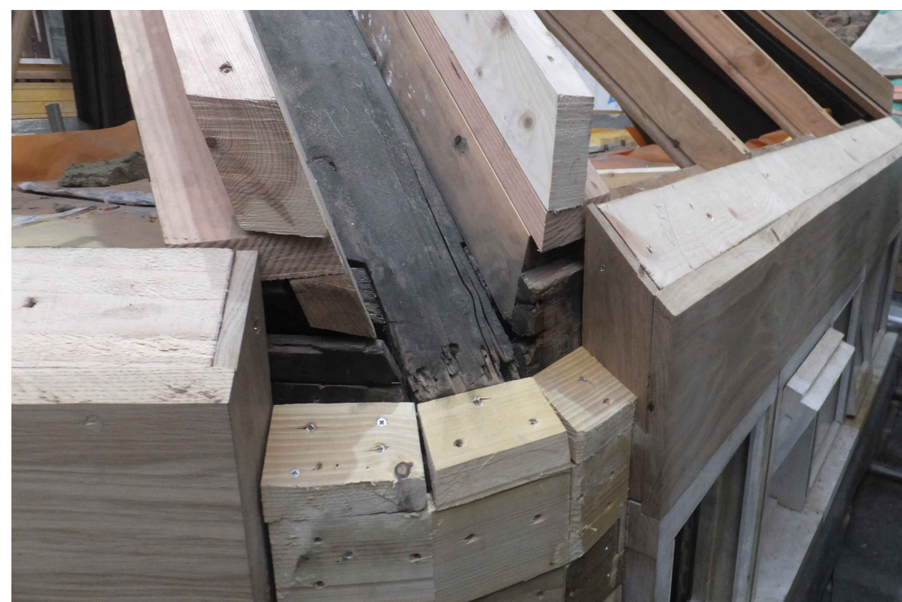
EXISTING EAVES OF VALLEY GUTTER
