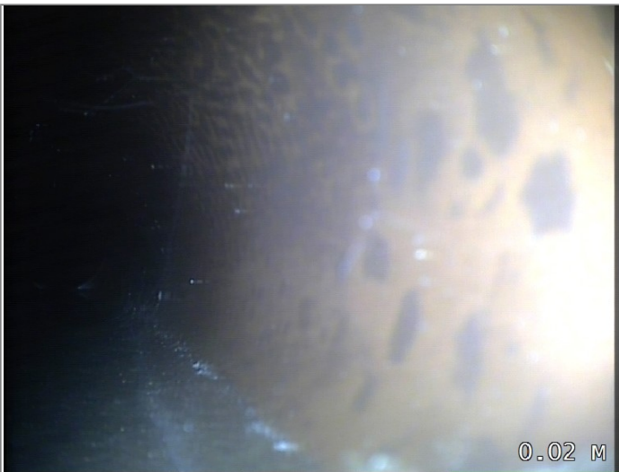
Start node type, manhole, reference MH05
