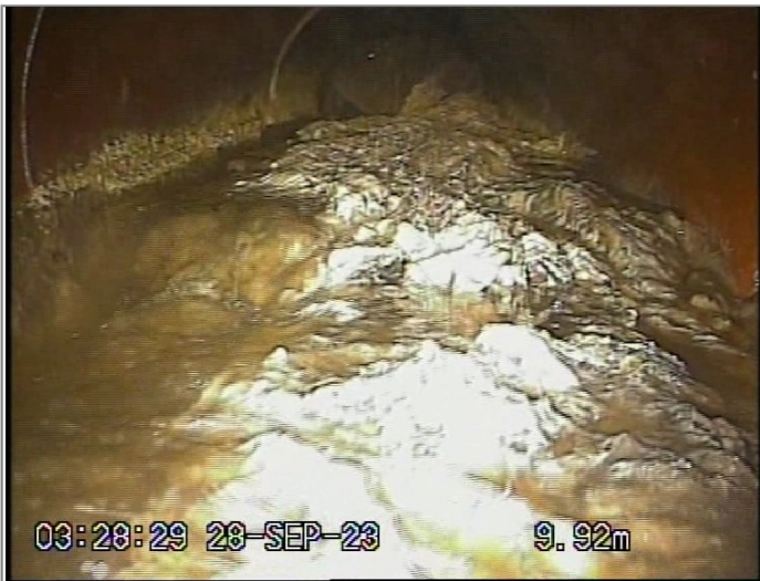
Other settled deposits 10% cross-sectional area loss - Remark: FOUL WASTE, Finished
