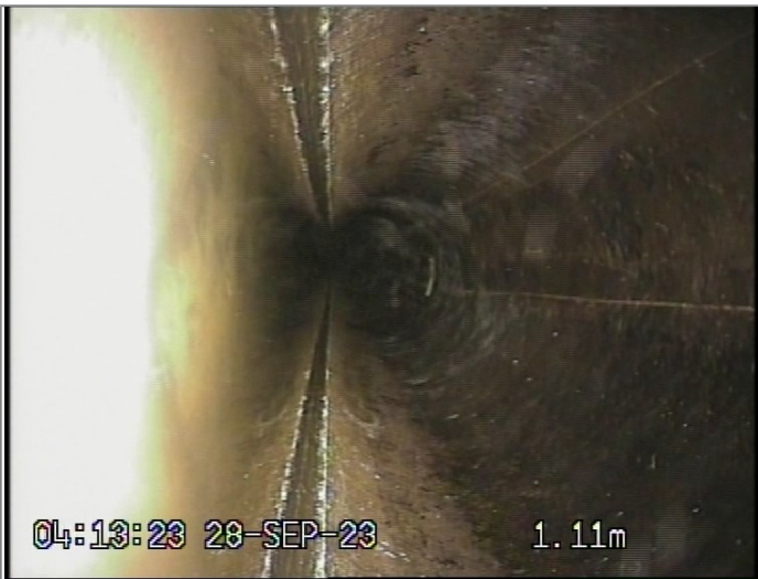
Point repair, pipe replaced from 12 to 12 o'clock
