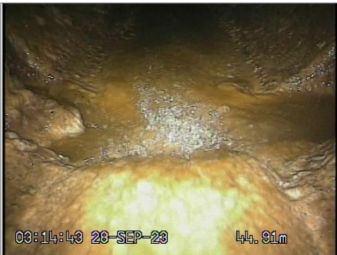
Open joint large
