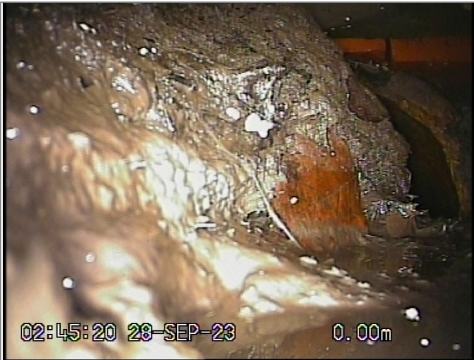
Start node type, manhole, reference MH 02
