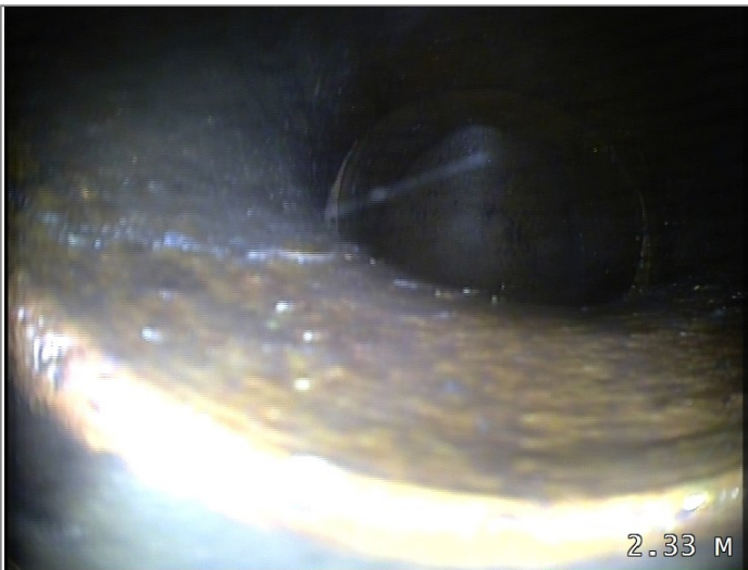
Start node type, manhole, reference MH01
