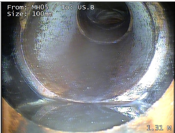
Open joint large
