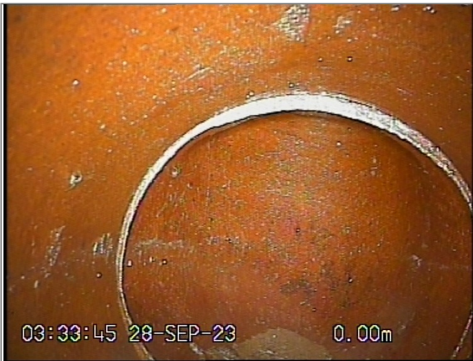
Start node type, manhole, reference UU 1203
