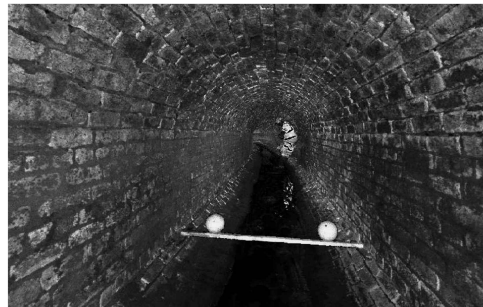
Figure 2.7 – Typical Section of Brick Barrel Culvert
