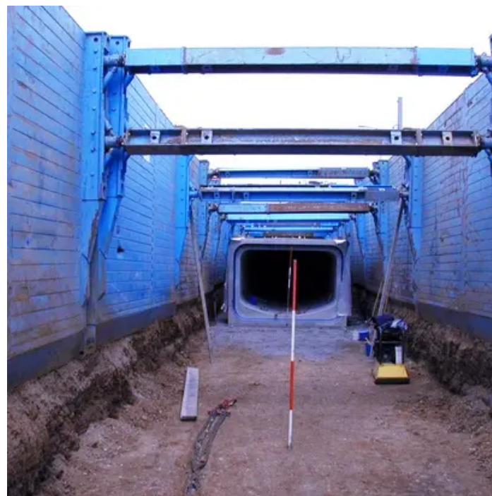
Figure 5.5 – Culvert Installation with Trench Boxes
