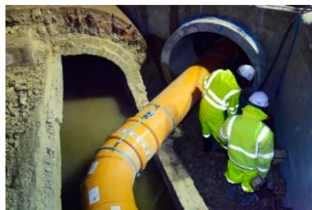
Figure 5.3 – Temporary Diversion of Flow
