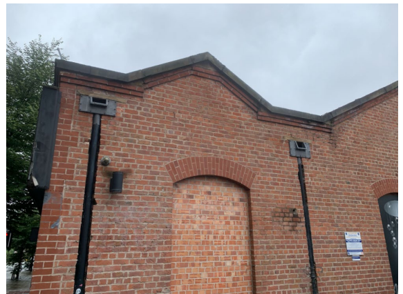
Picture 6 – Southeastern corner aspect
