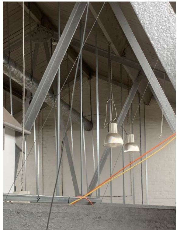
Picture 18 – Northern warehouse roof space
