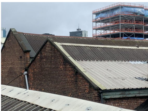
Picture 11 – Central pitched roofs
