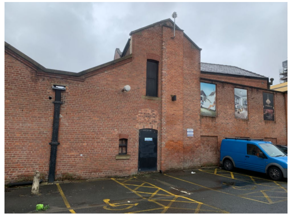
Picture 4 – Eastern aspect & pitched roof
