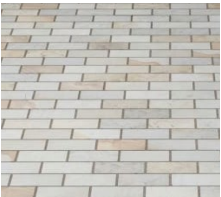
Sandstone paving to main routes
