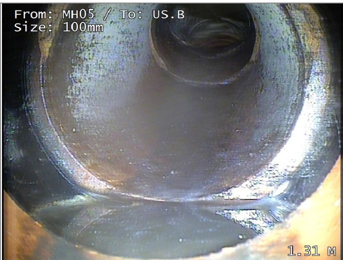
Open joint large
