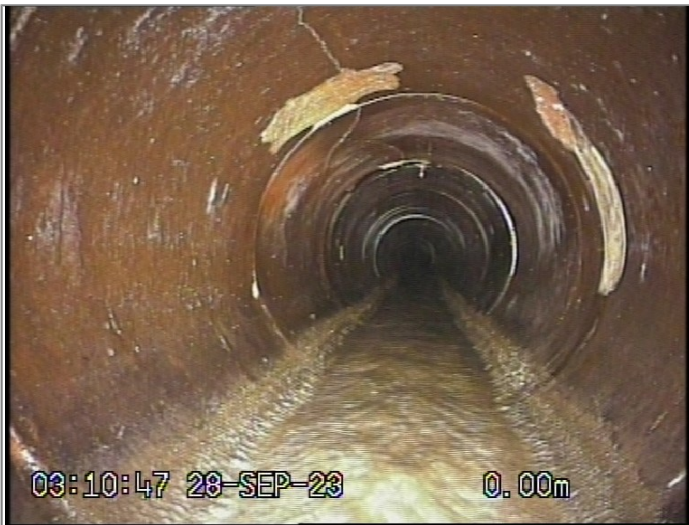
Start node type, manhole, reference UU 1204
