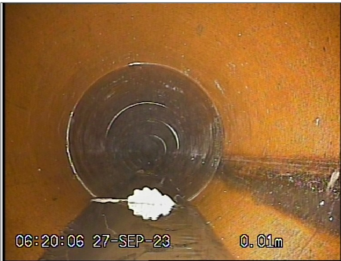
Start node type, manhole, reference UU 1202
