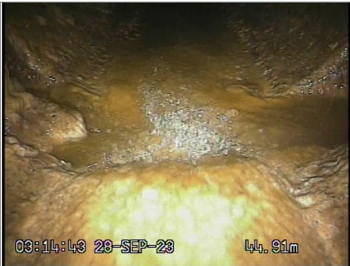
Open joint large
