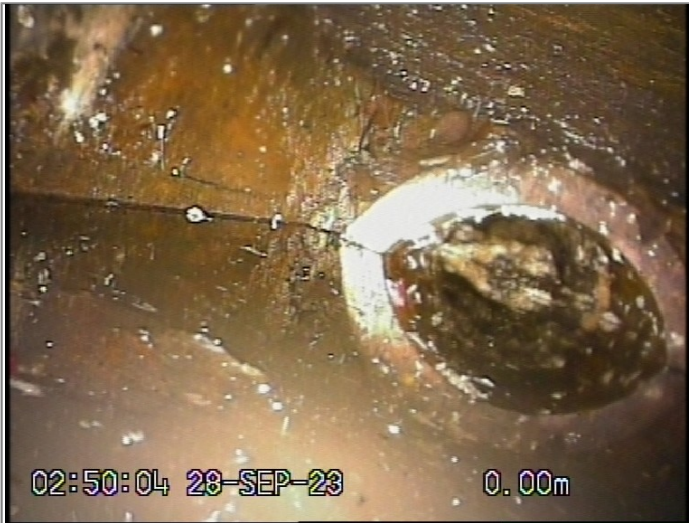
Start node type, manhole, reference MH 02
