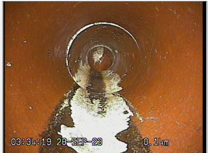
Finish node type, other special chamber, reference INTERNAL BACKDROP
