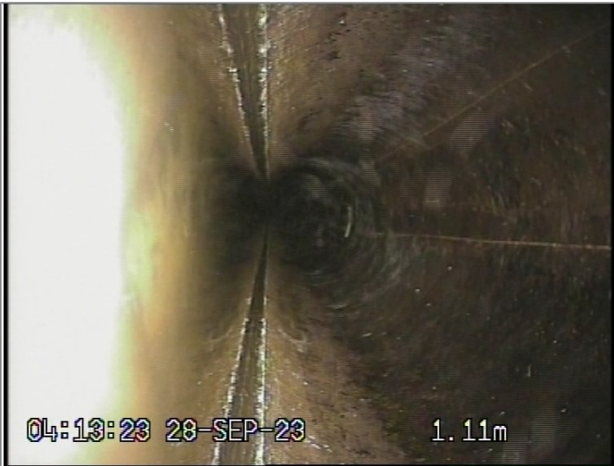
Point repair, pipe replaced from 12 to 12 o'clock
