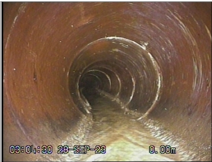
Start node type, manhole, reference UU 1203
