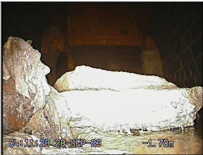
Start node type, manhole, reference UU 1201
