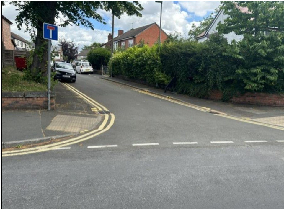
View of recently installed double yellow lines at the Ansleigh Avenue/Crumpsall Lane junction
