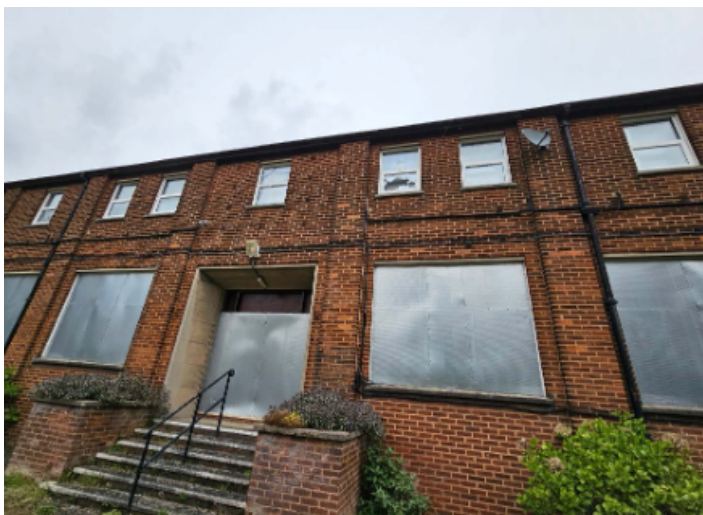
Views of existing building
