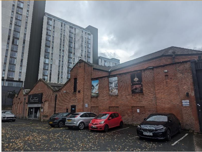
Photograph 1: The primary site building exterior
