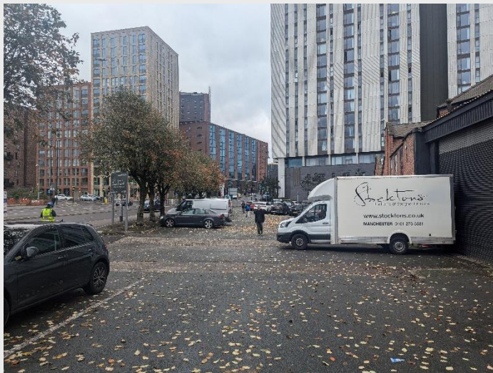
Photograph 3: Site carpark and tree row
