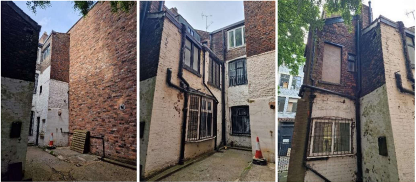
Figure 7 – Existing photographs of rear/side projections
