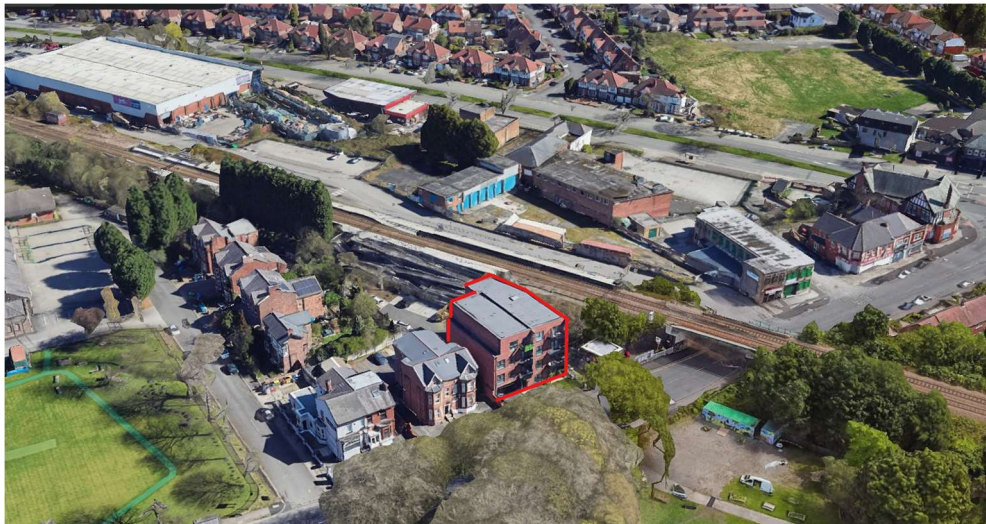
The four storey apartment building at 177 Mauldeth Road – edged red
