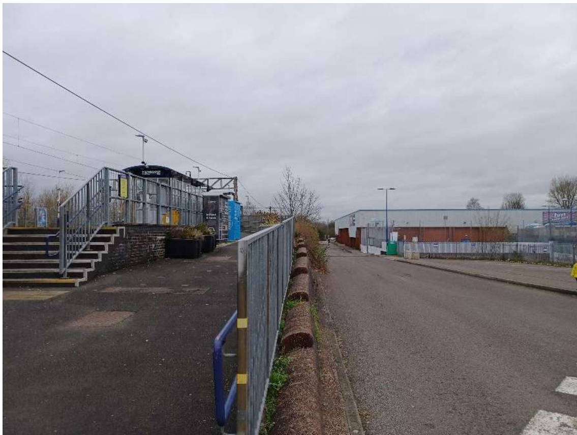
View north along the access road with the existing B and M Store to the right and Mauldeth Road train station southbound platform to the left
