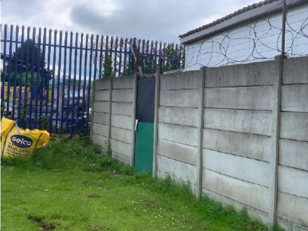
P9: Fenced off building located in the south-eastern corner of the site
