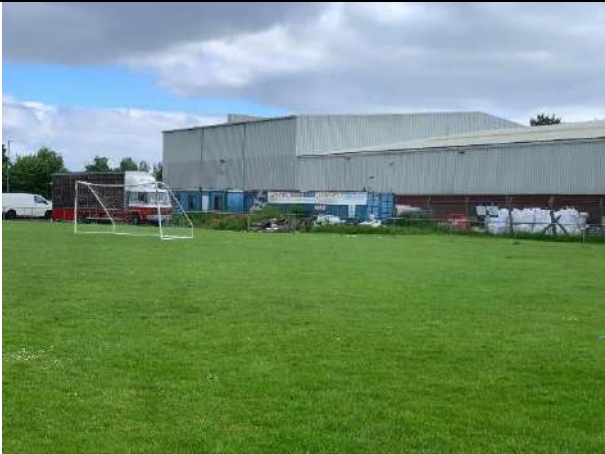
P2: View of the site from towards the south-western corner facing east
