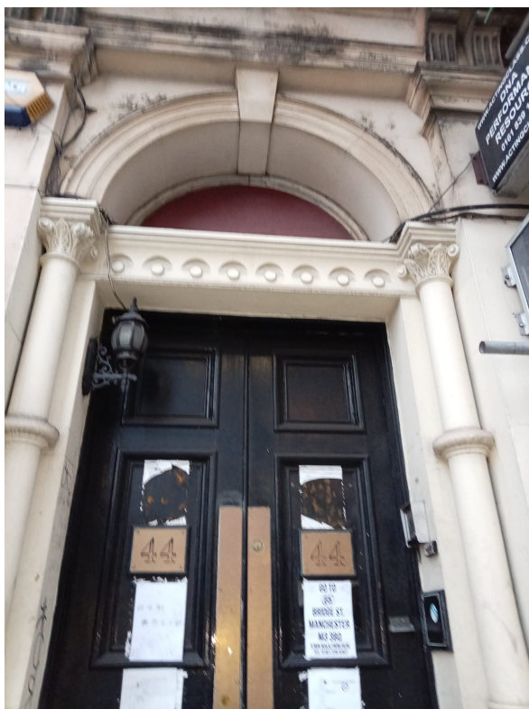
Photo 6 – Entrance door right hand side
