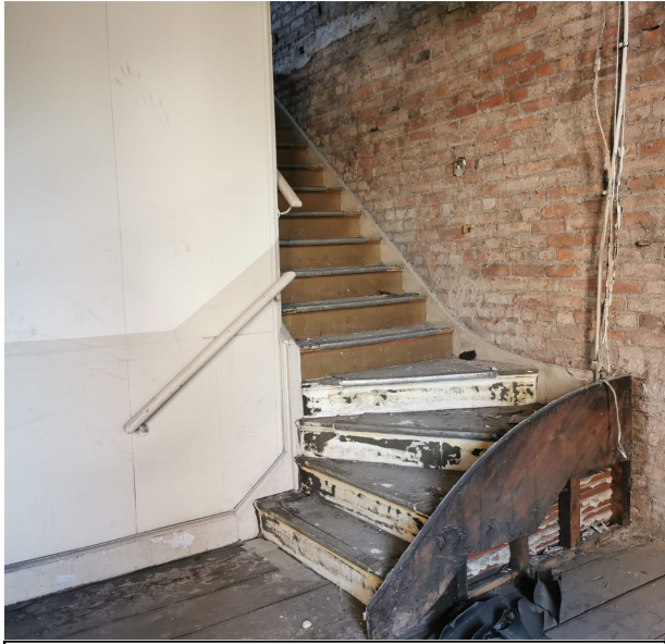
Photo 29 – Main stair to upper floors with the lift shaft.
