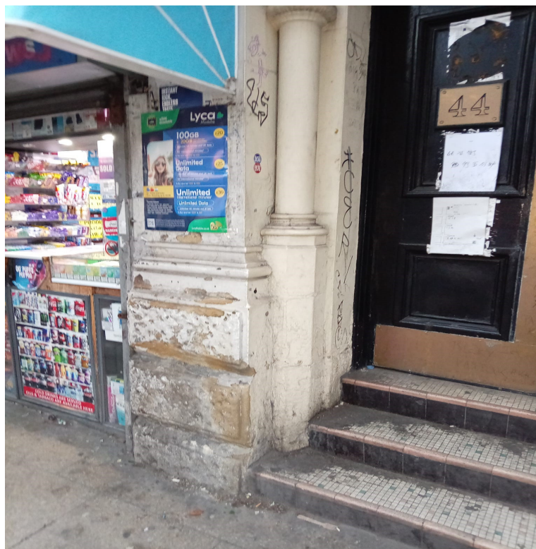
Photo 8 – Kiosk with the canopy, entrance door on the right side with 3 steps
