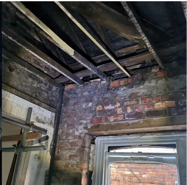
Photo 20 – 4 th floor part of the roof void
