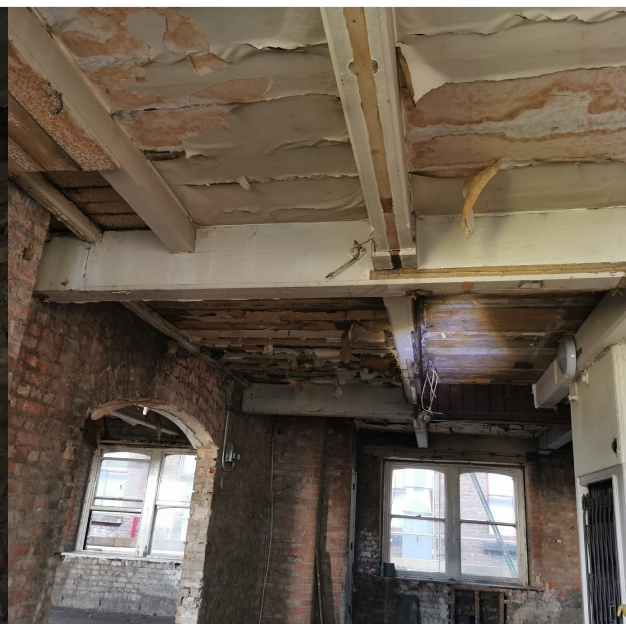
Photo 39 – 2 nd floor windows facing to the rear and showing the existing timber beams and timber boards and cross walls
