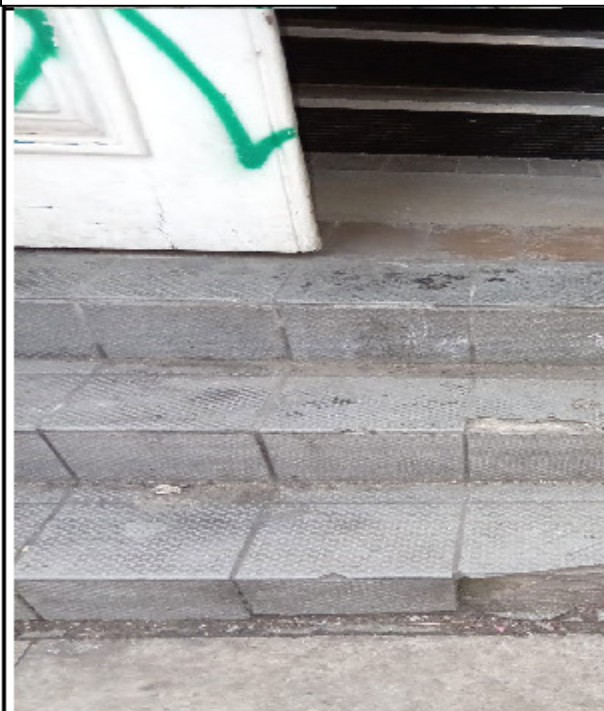
Photo 3 entrance door steps Left side
