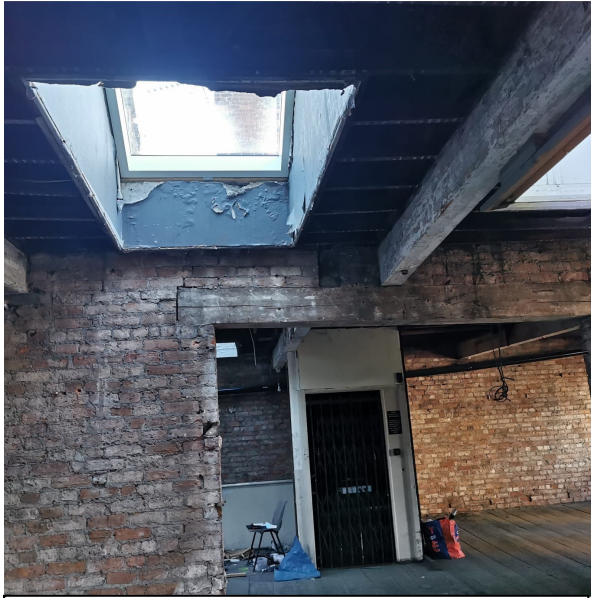
Photo 17 – 4 th floor skylights and fire exit
