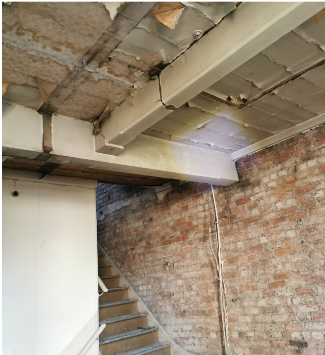
Photo 31 – Main stair showing the existing timber beams First floor level
