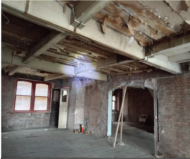
Photo 33 – 3 rd floor windows facing to the rear and showing the existing timber beams and cross walls
