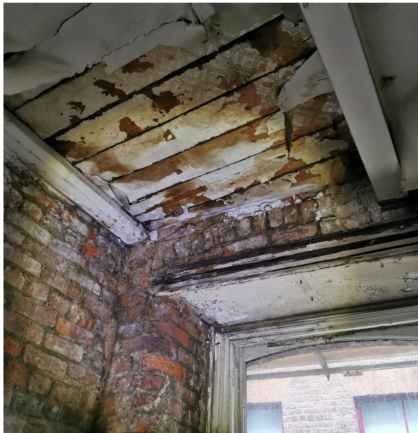
Photo 36 – 2 nd floor windows facing to the rear and showing the existing timber beams and timber boards
