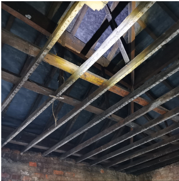
Photo 27 – 4 th floor timber roof truss
