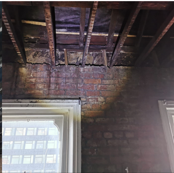
Photo 28 – 4 th floor front windows and part of the roof void
