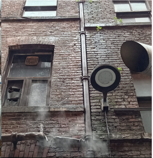
Photo 10 – Rear Elevation First floor windows
