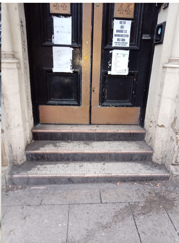
Photo 7 – Entrance door right hand side with steps
