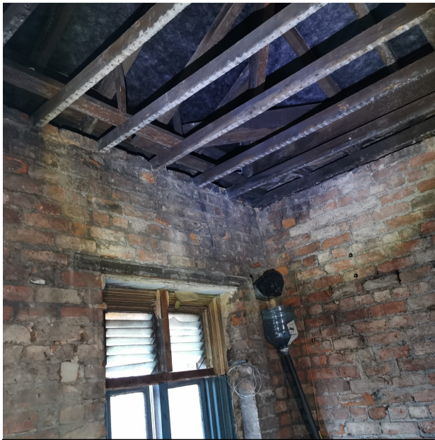
Photo 23 – 4 th floor window facing to Reyner Street and part of the roof void
