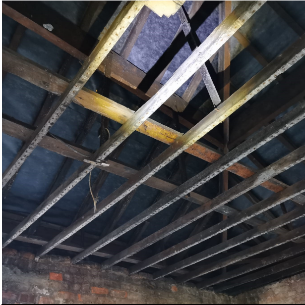
Photo 21 – 4 th floor part of the roof void
