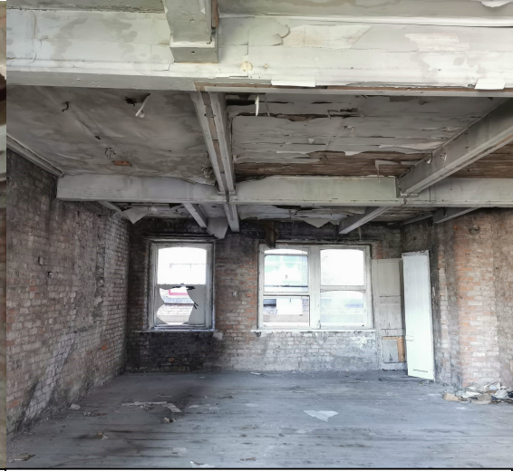
Photo 34 – 3 rd floor windows facing to the rear and showing the existing timber beams
