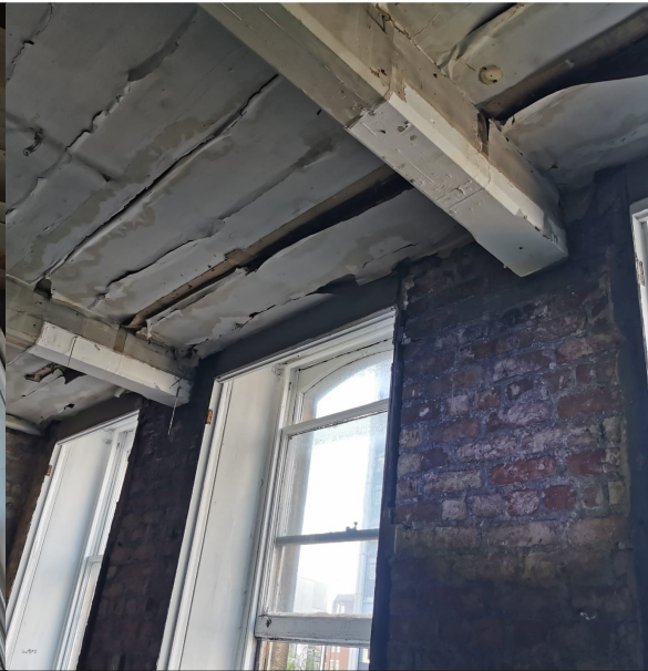
Photo 35 – 3 rd floor windows facing to the front and showing the existing timber beams
