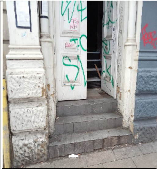
Photo 4 entrance double panel door Left side with steps
