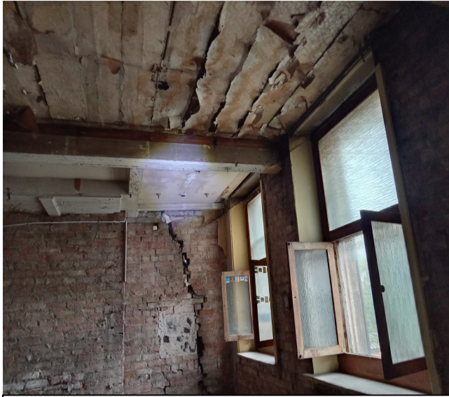
Photo 40 – First floor windows facing to the front and showing the existing timber beams and timber boards
