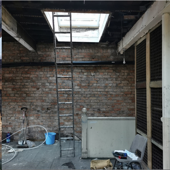
Photo 18 – 4 th floor skylights
