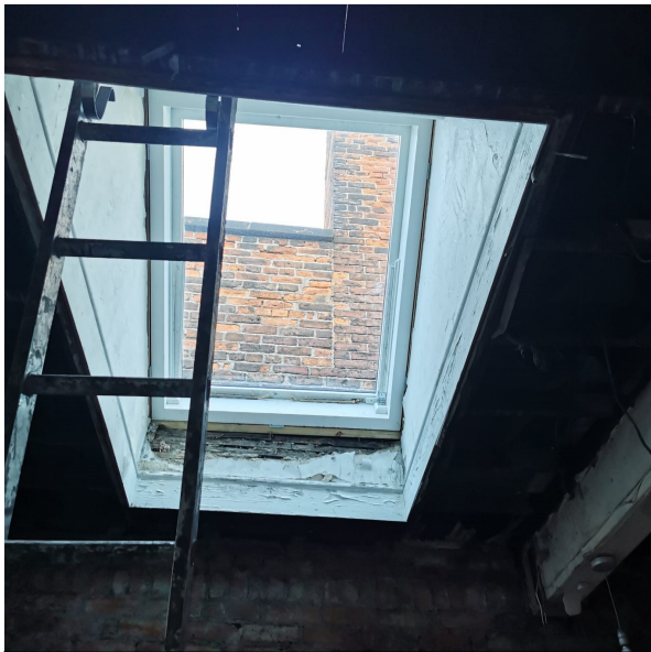
Photo 19 – 4 th floor skylight
