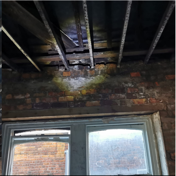
Photo 22 – 4 th floor window and part of the roof void
