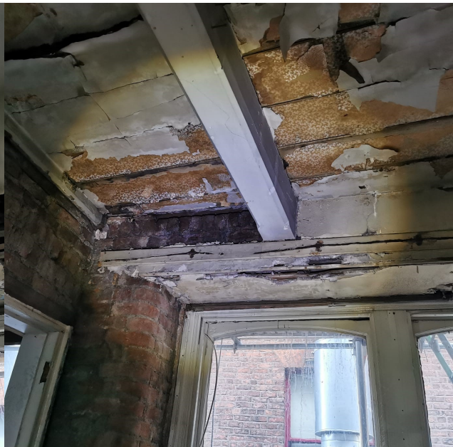
Photo 37 – 2 nd floor windows facing to the rear and showing the existing timber beams and timber boards
