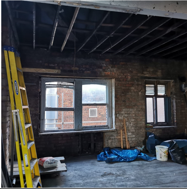
Photo 13 – 4 th floor windows facing Reyner Street
