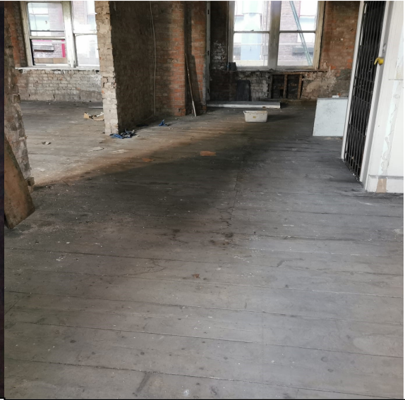
Photo 41 – First floor windows facing to the rear and showing the existing timber boards
