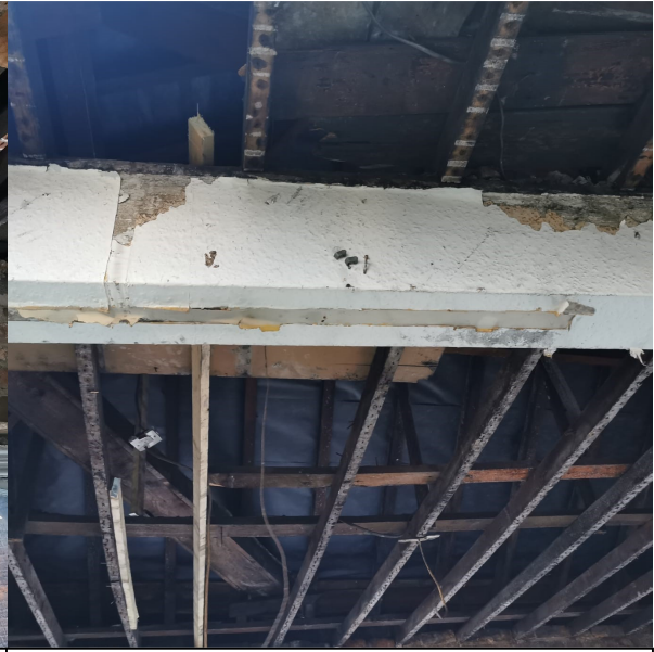
Photo 26 – 4 th floor timber roof truss
