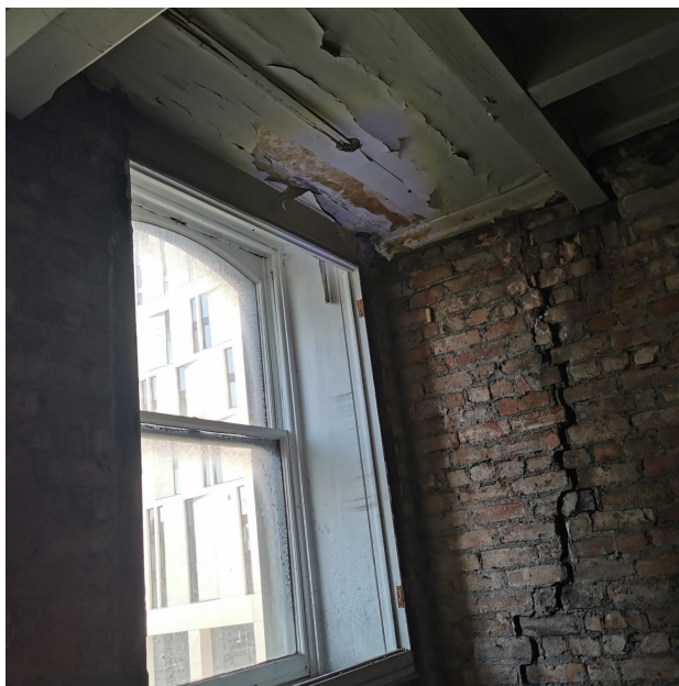
Photo 38 – 2 nd floor windows facing to the front and showing the existing timber beams and timber boards and cross walls
