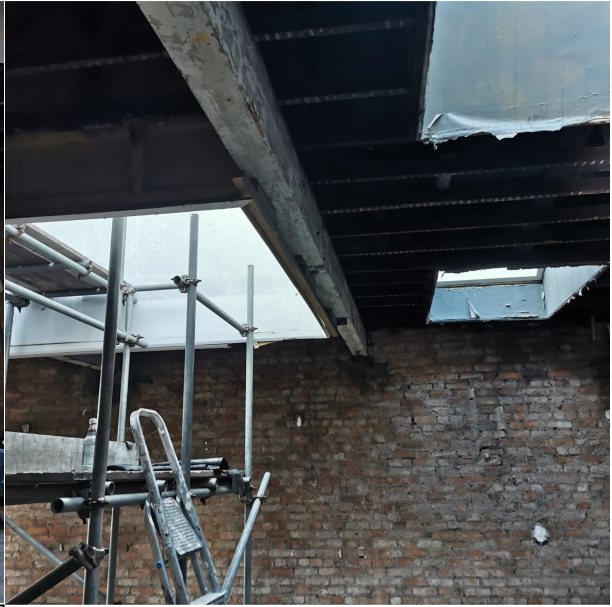
Photo 14 – 4 th floor skylights
