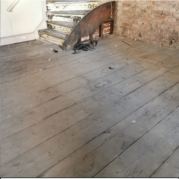
Photo 30 – Main stair showing the existing timber floor boards
