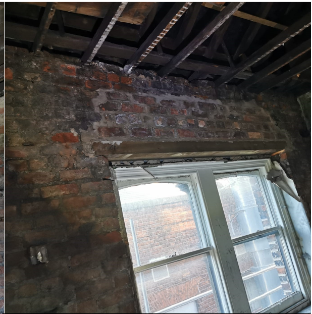
Photo 24 – 4 th floor window facing to Reyner st. and part of the roof void
