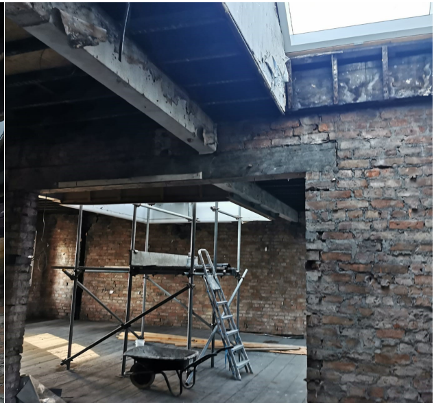
Photo 16 – 4 th floor skylights
