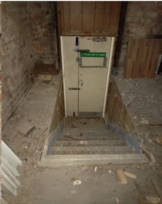
Photo 32 – Fire exit door to Reyner Street Upper Ground level
