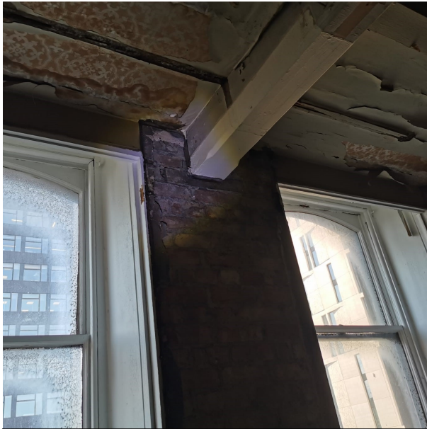
Photo 34 – 3 rd floor windows facing to the front and showing the existing timber beams
