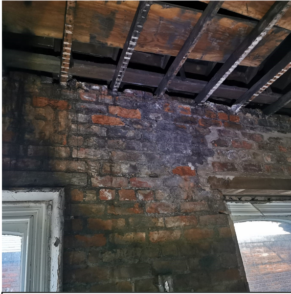
Photo 25 – 4 th floor rear windows and part of the roof void
