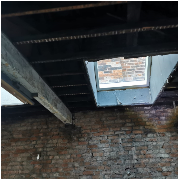
Photo 15 – 4 th floor skylights
