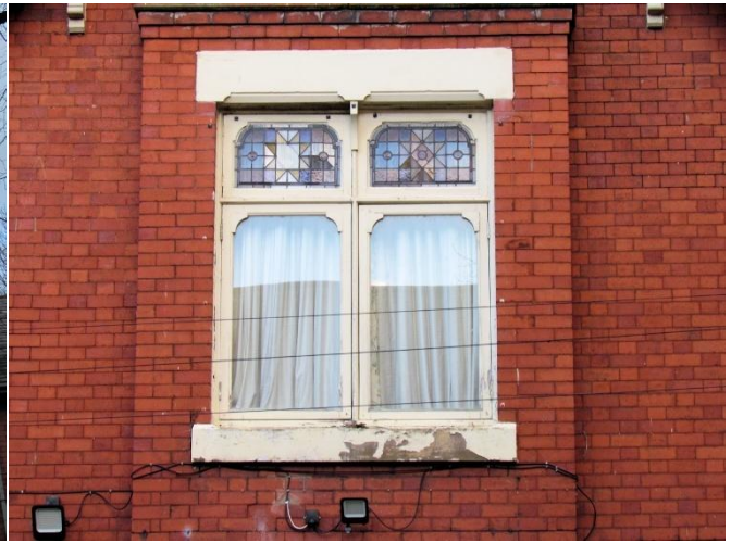
Detail of First-floor Window
