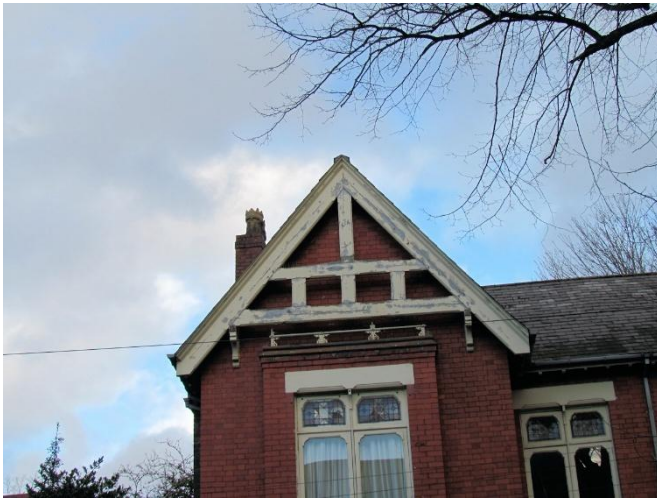
Detail of Gable
