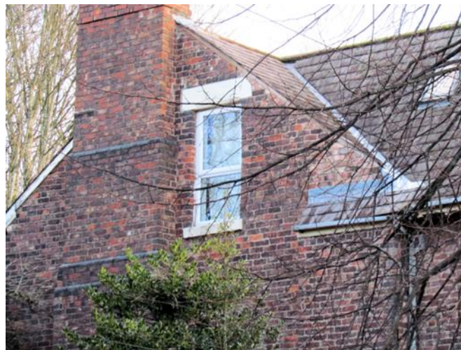
Gable of West Elevation
