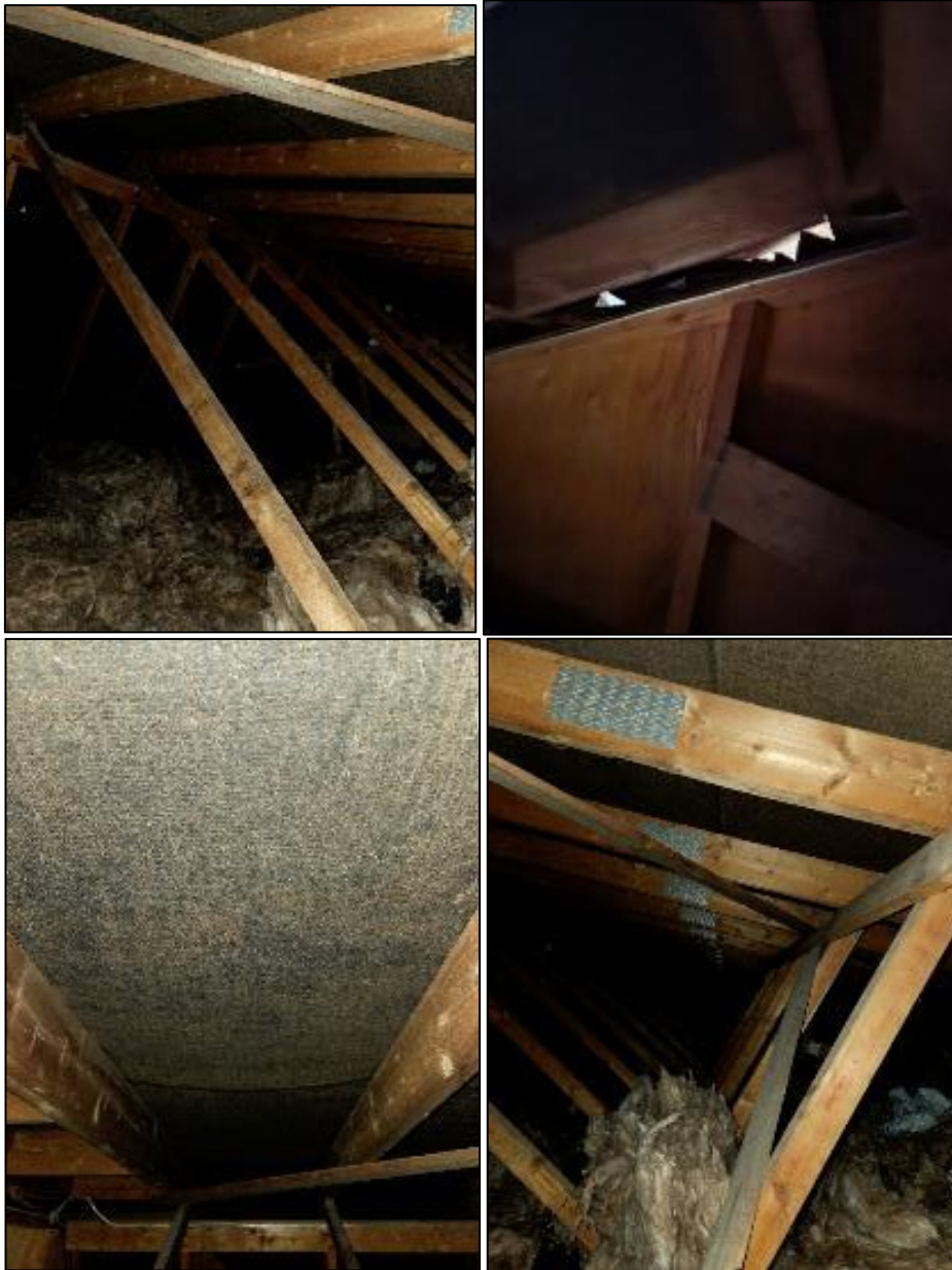
Photograph 9 (top left), 10 (top right), 11 (bottom left) & 12 (bottom right) showing the internal roof void
