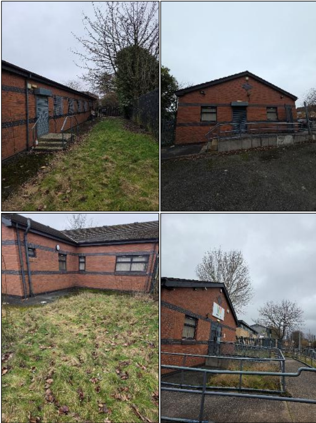
Photograph 1 (top left), 2 (top right), 3 (bottom left) & 4 (bottom right) showing the exterior of B1
