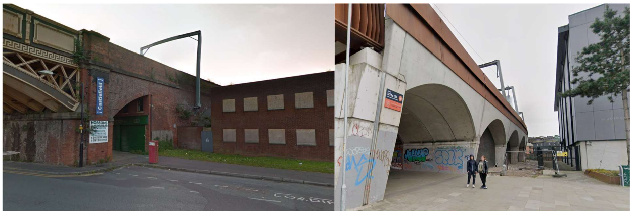
Rear of application site as seen from Water Street in 2014 (Left) and in 2025 (Right)
