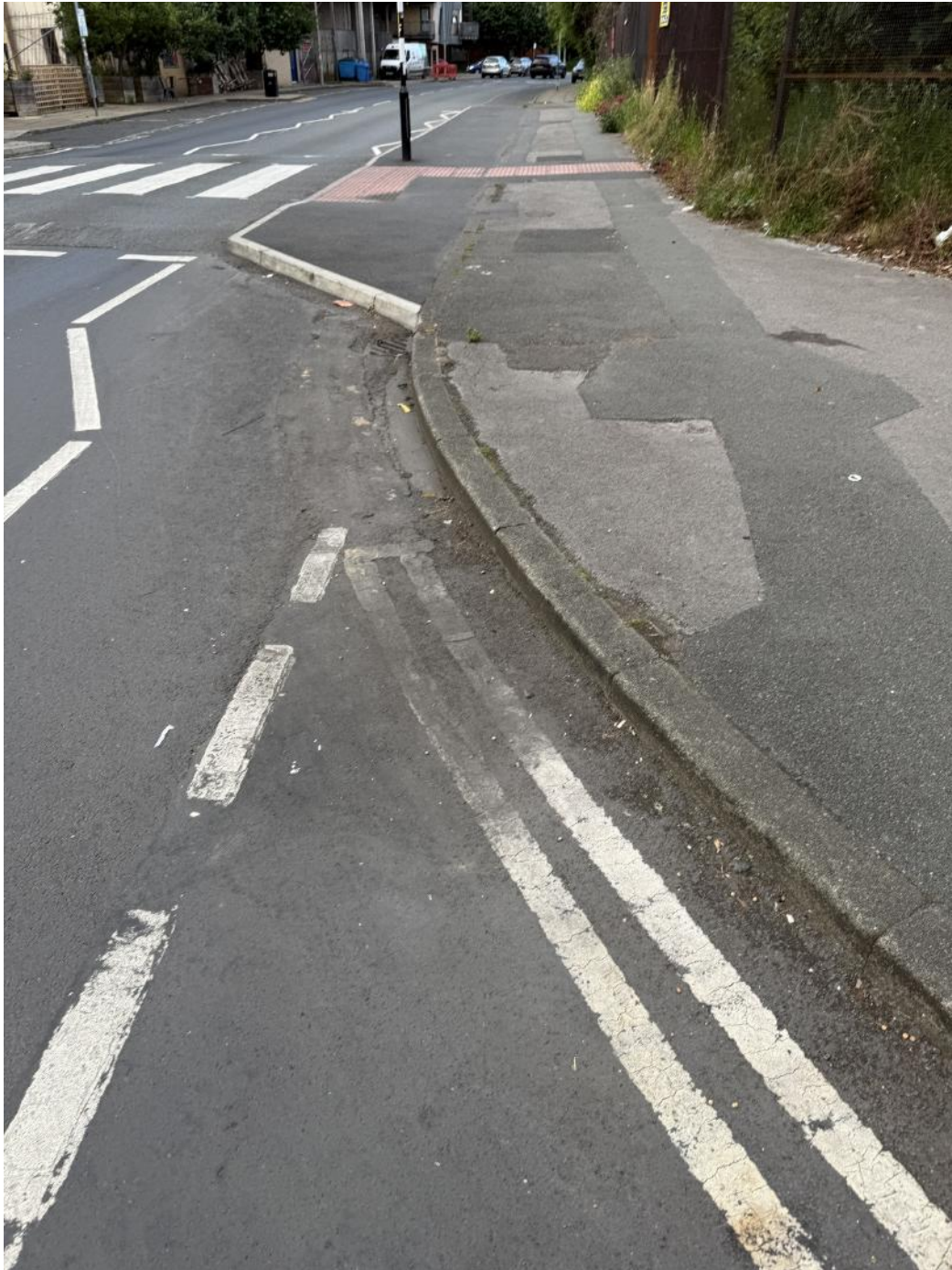
Tarmac Patch repairs.
