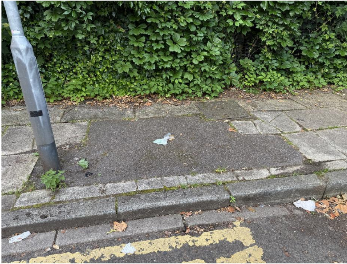
Tarmac patch repair in concrete slabbed footpath.
