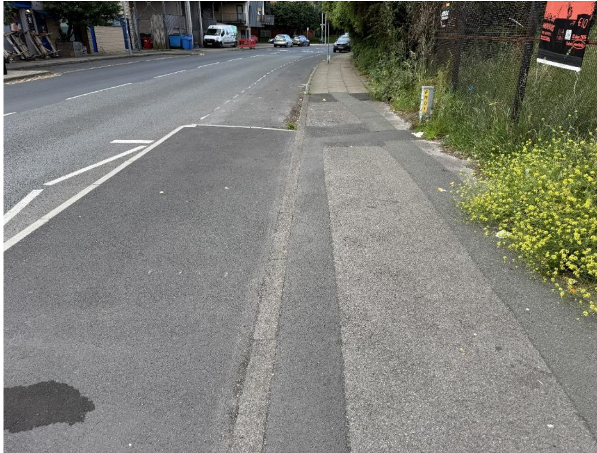
Overview of footpath.
