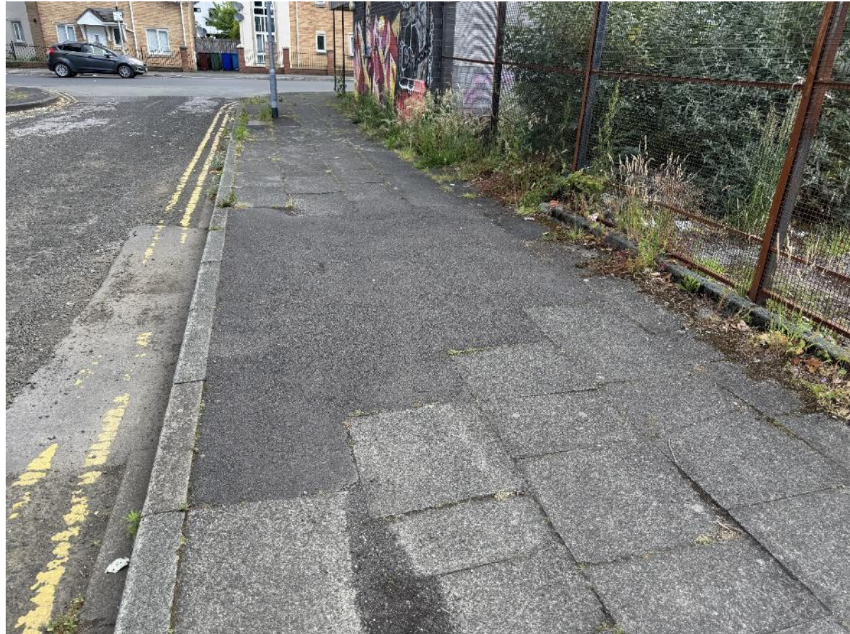
Tarmac patch repair in concrete flagged footpath.
