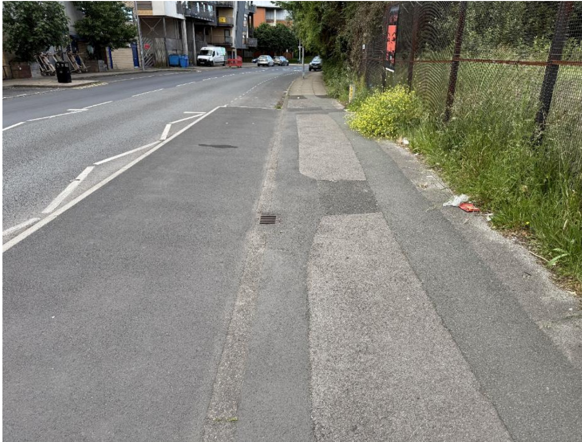
Tarmac patch repairs and gully in footpath.
