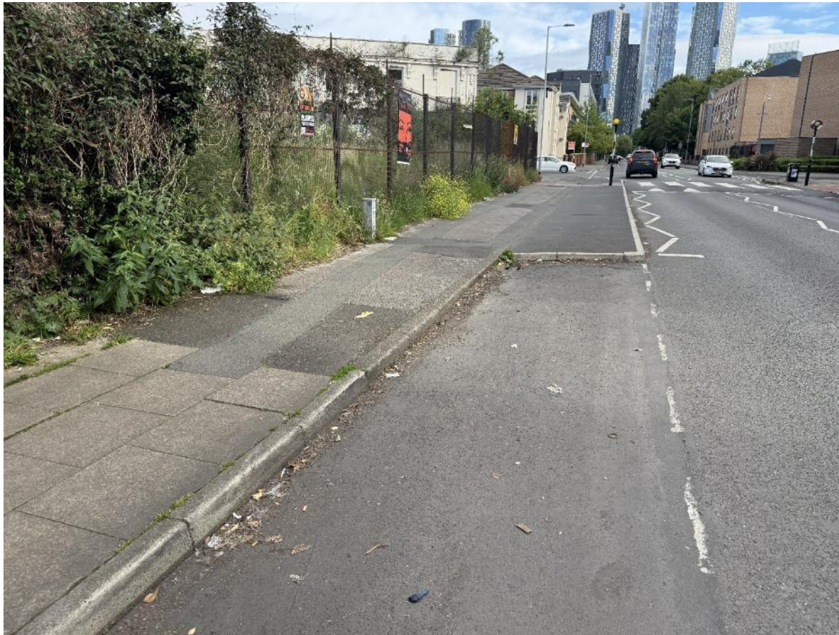
Overview of footpath.
