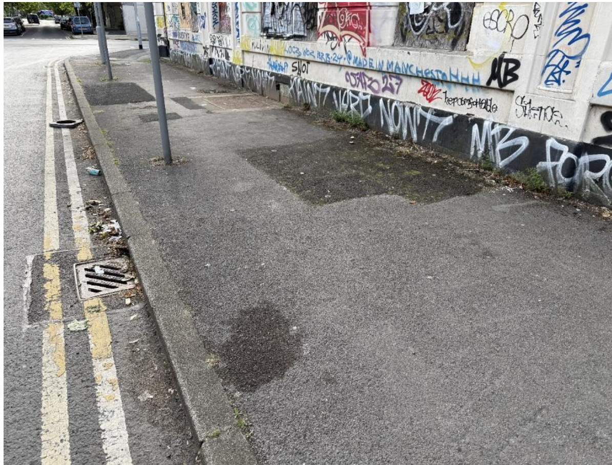
Patch repairs in tarmac.
