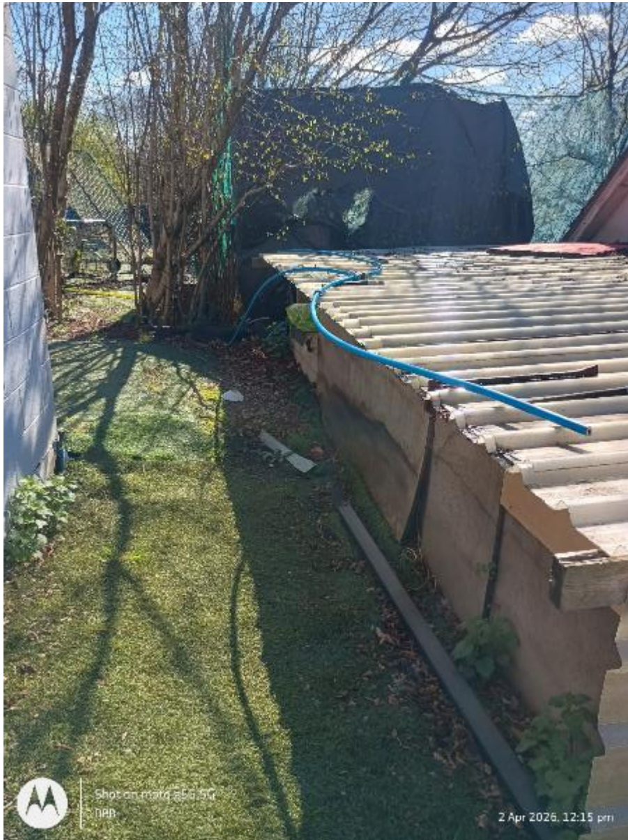
Roof of existing outhouse with T1 group Hazels (above)
