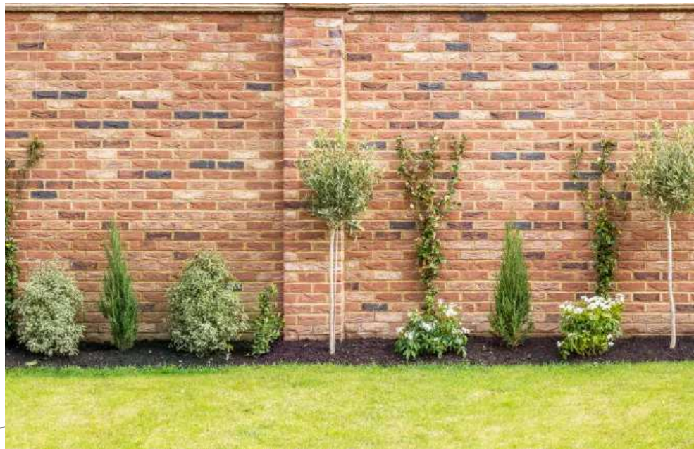
EXISTING BRICK GARDEN WALL
