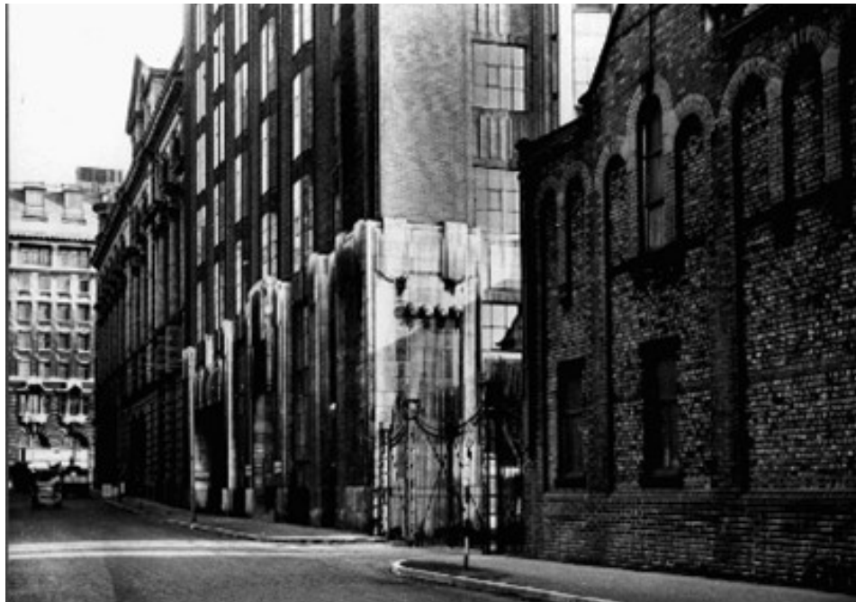
Figure 16 No.90 Great Bridgewater Street (Lee House) with No.56 Oxford Street (former Tootal Building) attached. View looking towards Oxford Street from Great Bridgewater Street. Photo dated 1965. Image courtesy of Manchester Libraries.
