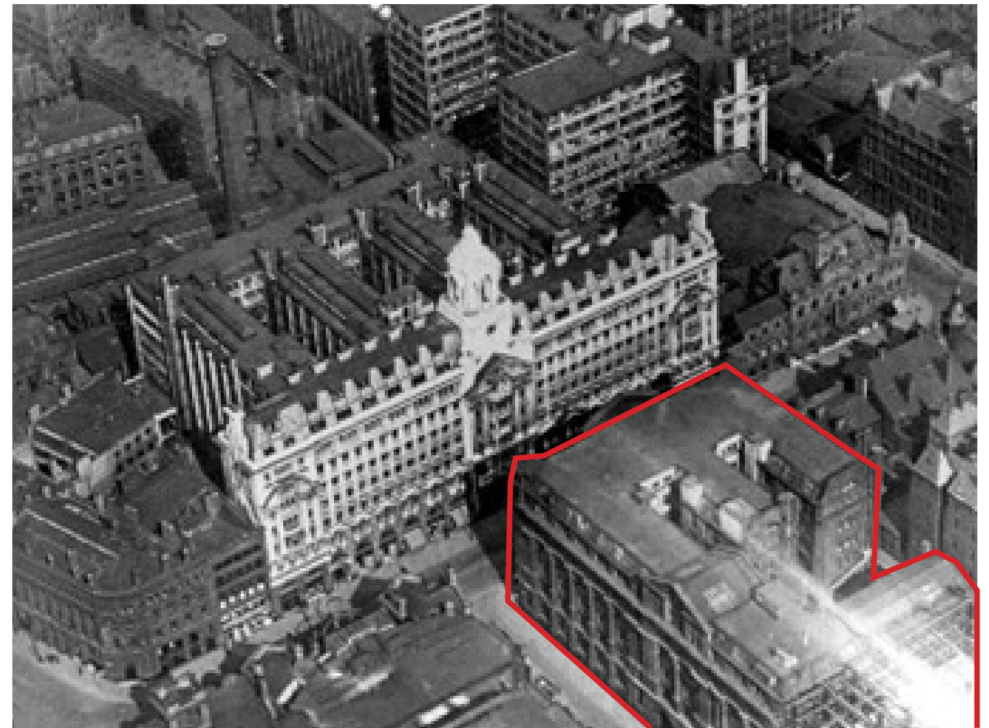
Figure 09 No.56 Oxford Street in bottom right of image. - Aerial view with No.90 Great Bridgewater Street (Lee House) under construction. Steel structure visible in bottom right of photograph. Photo dated 1930. Image courtesy of Manchester Libraries.
