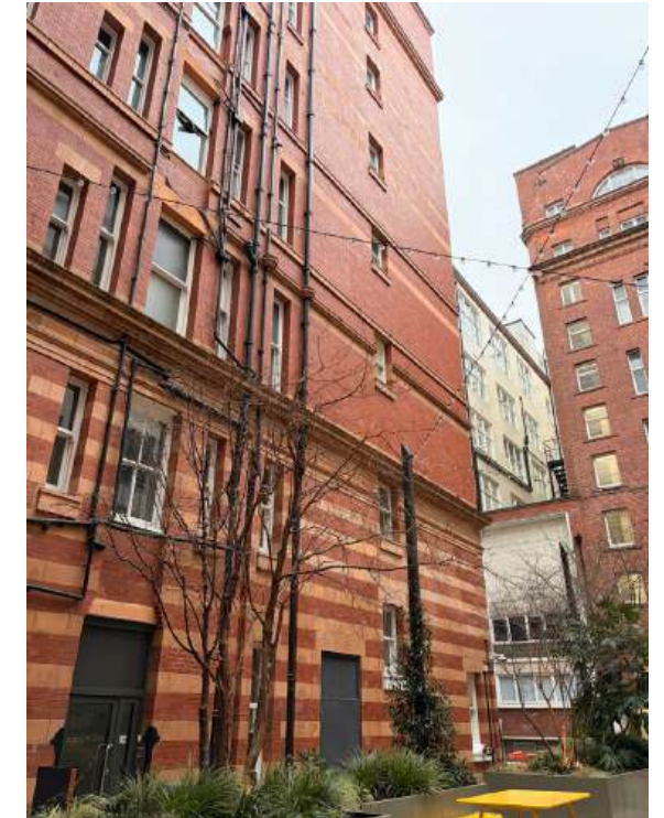
C View towards the rear of the Broadhurst House with the three storey infills dating from the 1960's
