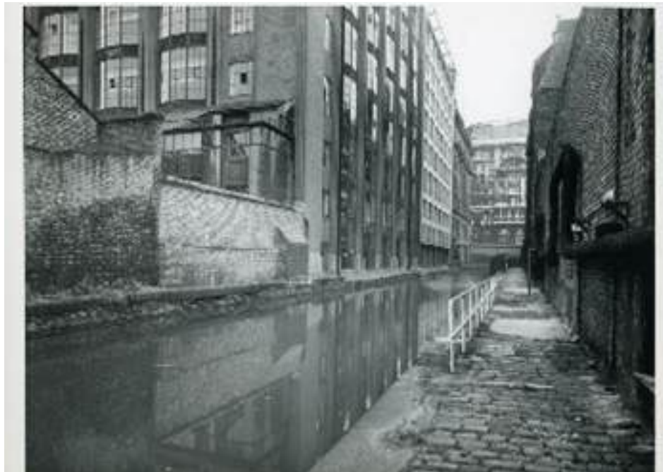
Figure 12 No.90 Great Bridgewater Street and No.56 Oxford Street. - Photograph from canal side with Lee House on left hand bank, 1960's infill block and No.56 Oxford Street beyond. St. James Buildings in distance on opposite side of Oxford Street. Photo dated 1964. / Image courtesy of Manchester Libraries
