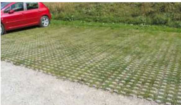
Permeable paving option for parking spaces.
