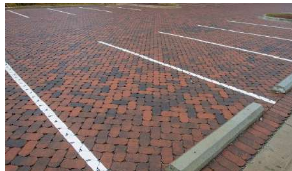
Extensive permeable paving for the whole road.
