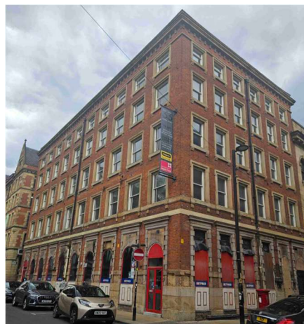
Application site as of April 2026.
