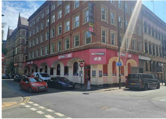
Application site as of June 2025.
