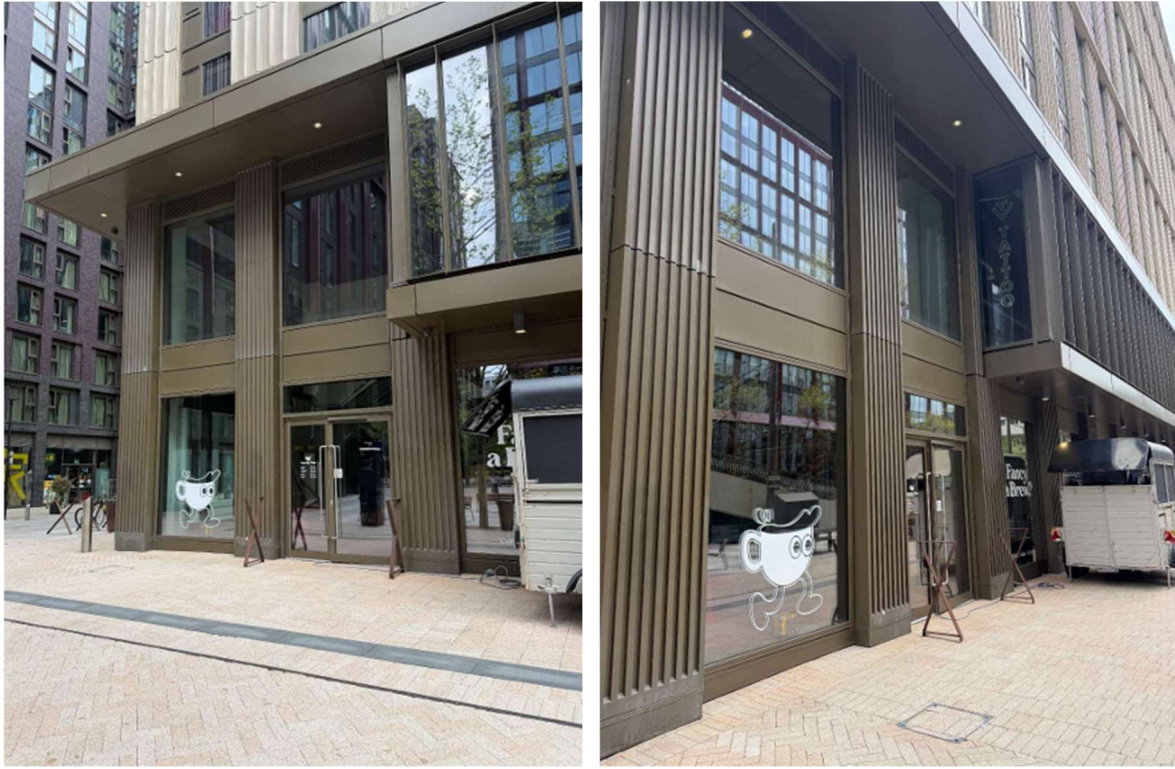
Front elevation of the ground and first floor
