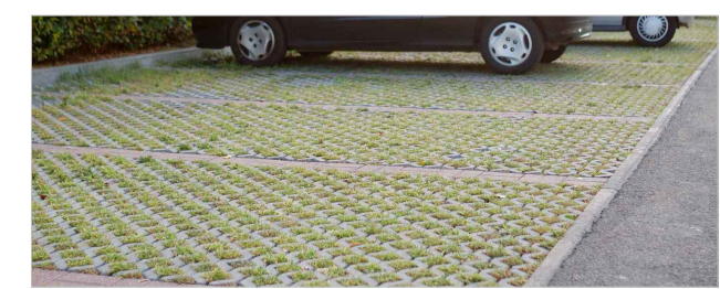
Permeable paving example
