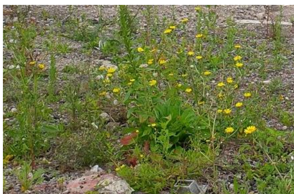
Figure 6—3 Typical brown roof – self-seeded brownfield habitat and mixed recycled substrate
