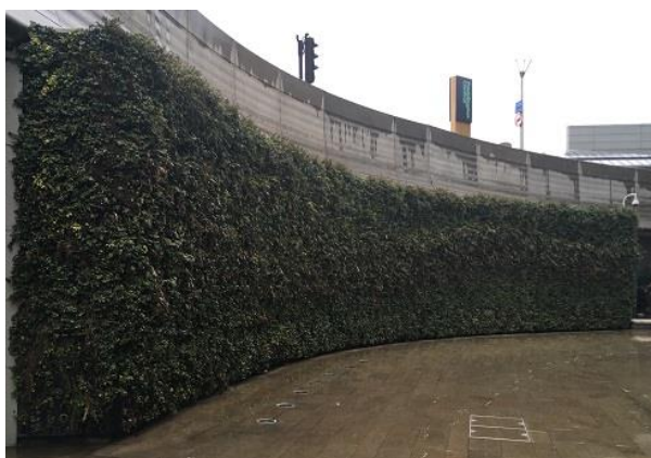
Figure 6—6 Modular green wall (Paddington, London)
