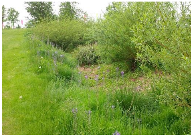
Figure 6—10 Vegetated conveyancing swale planted with native, pollen-rich species (Olympic Park, Stratford)
