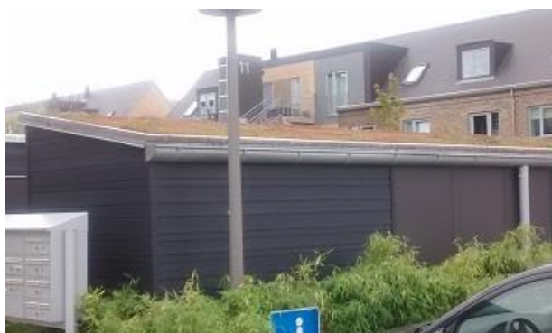
Figure 6—1 Extensive Sedum green roof above cycle store/garages (Nyborg, Denmark)
