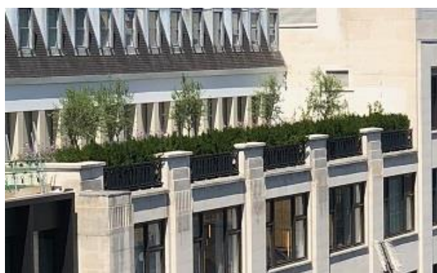
Figure 6—4 Intensive green roof (roof garden)(London)
