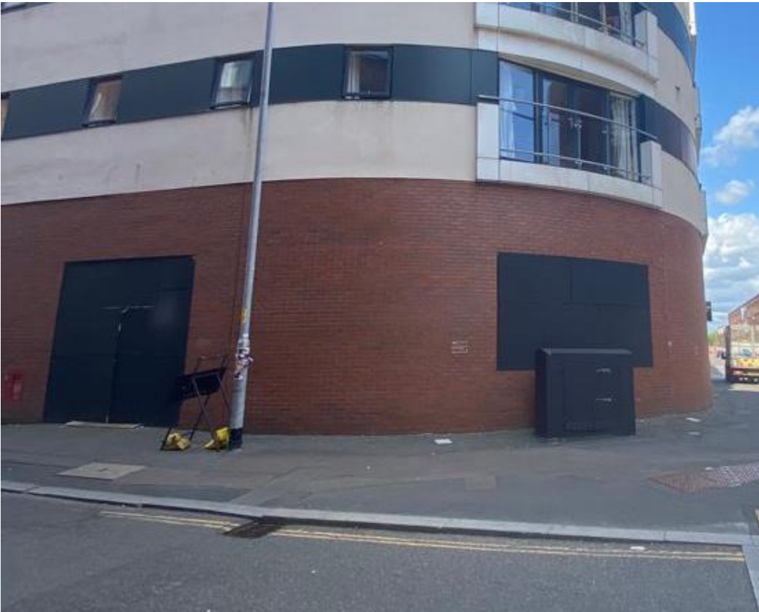
View B – Unit 49 Bengal Street
