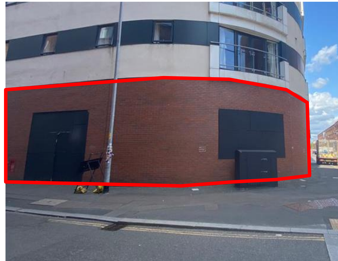
View from Jersey Street of Unit 2
