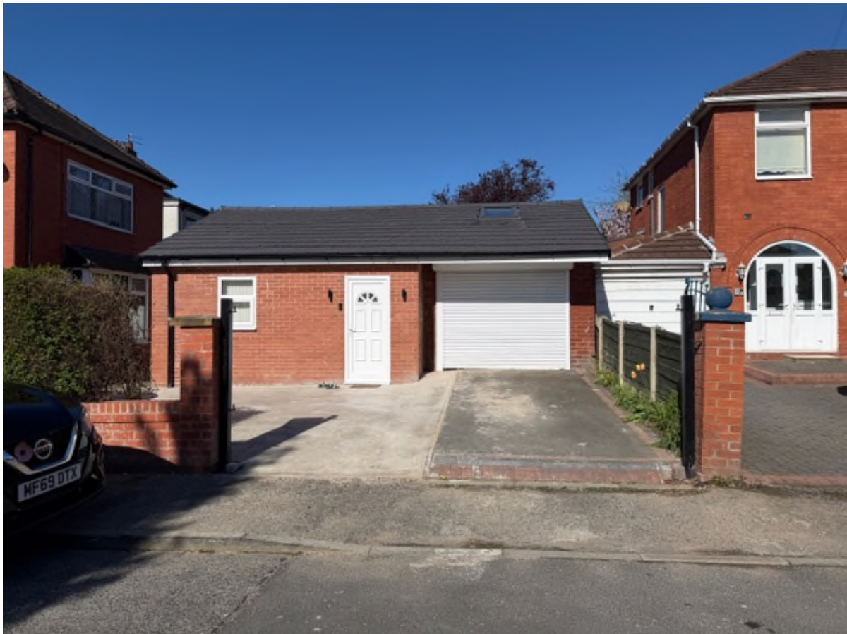
Figure 1: Front view of retrospective development from Kingston Grove
