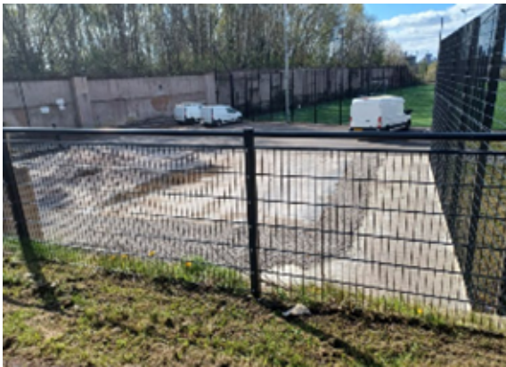
Site following demolition of the auto electrical workshop facing westwards
