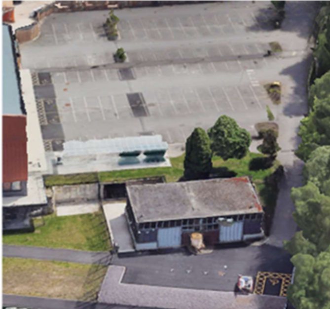
Visual looking eastwards with the former auto electrical workshop in the foreground.
