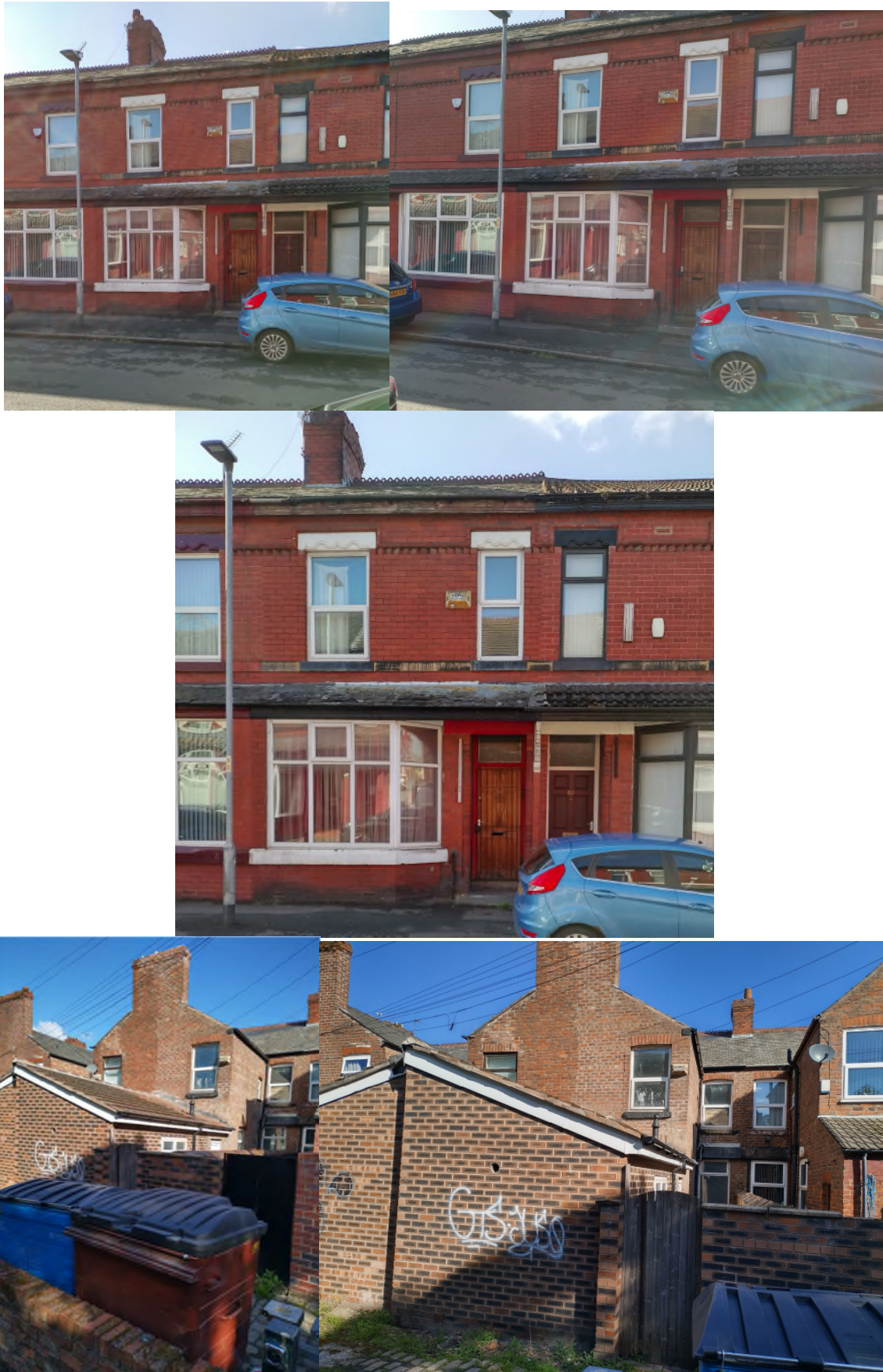
Fig.1 – Views of the front and rear of 22 Banff Road.
