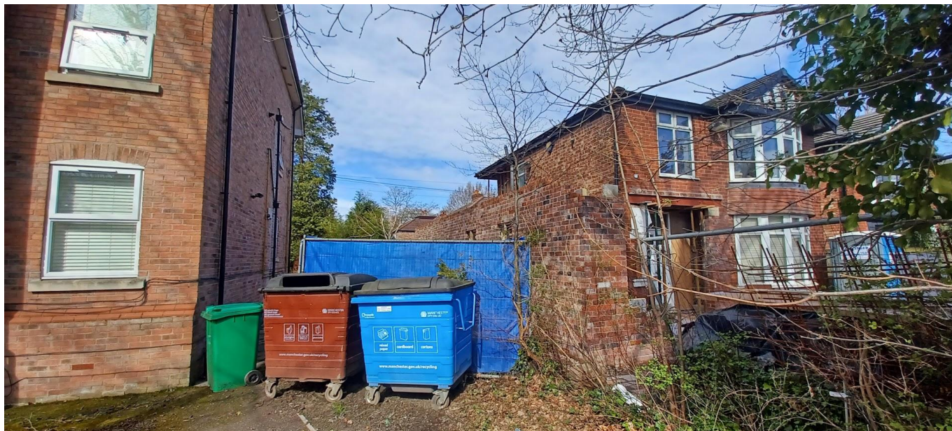
Site photograph (March 2026)
