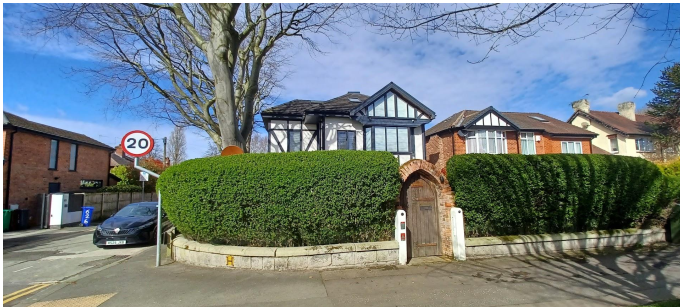
View of principal elevation of No.624 Wilmslow Road
