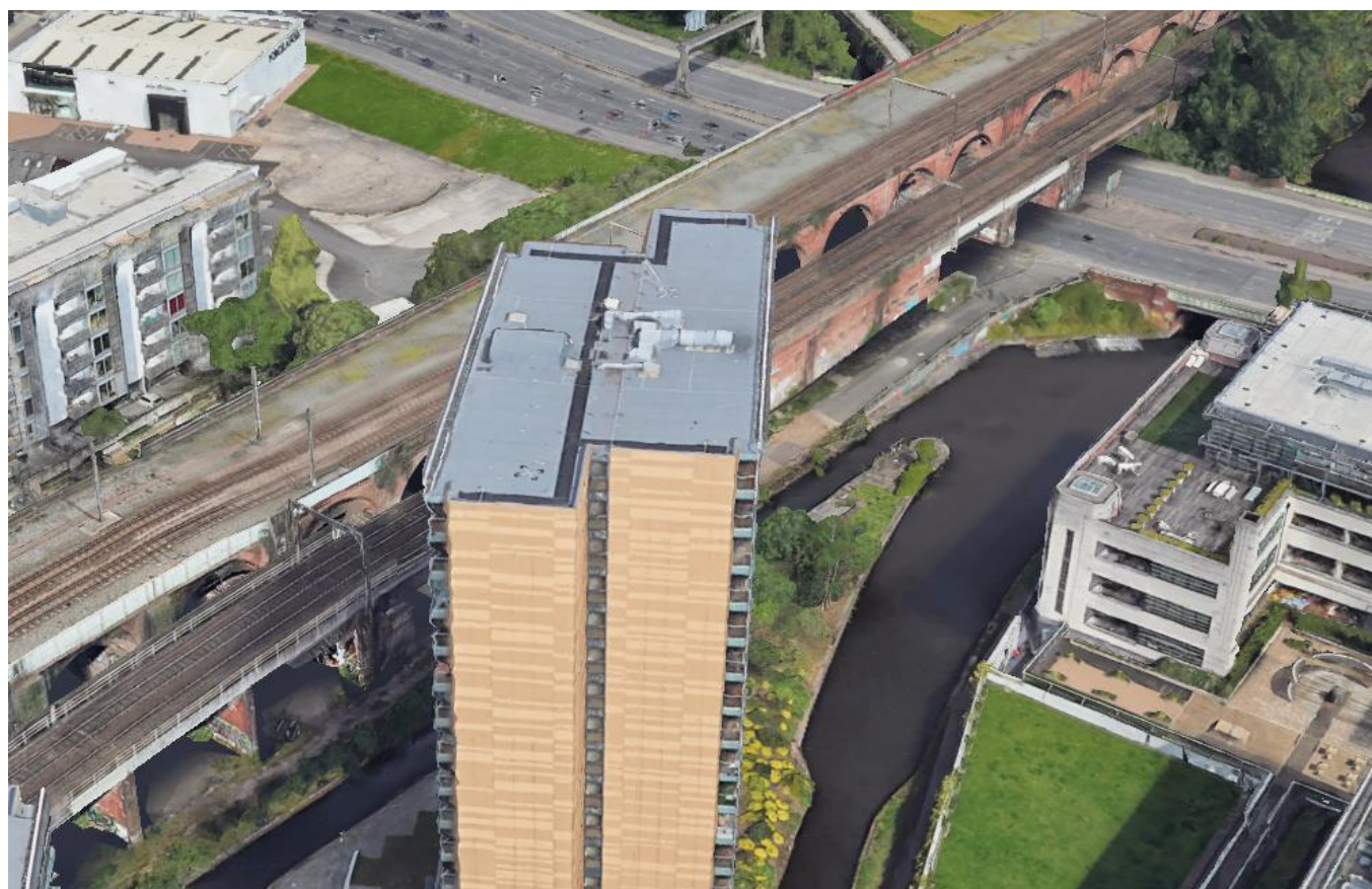
Google Earth capture of roof as it currently appears
