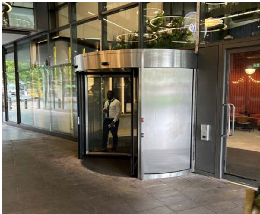
a defensive entrance featuring solid metal security shutters to revolving door; further security screens to the reception glazing; permanent security presence
