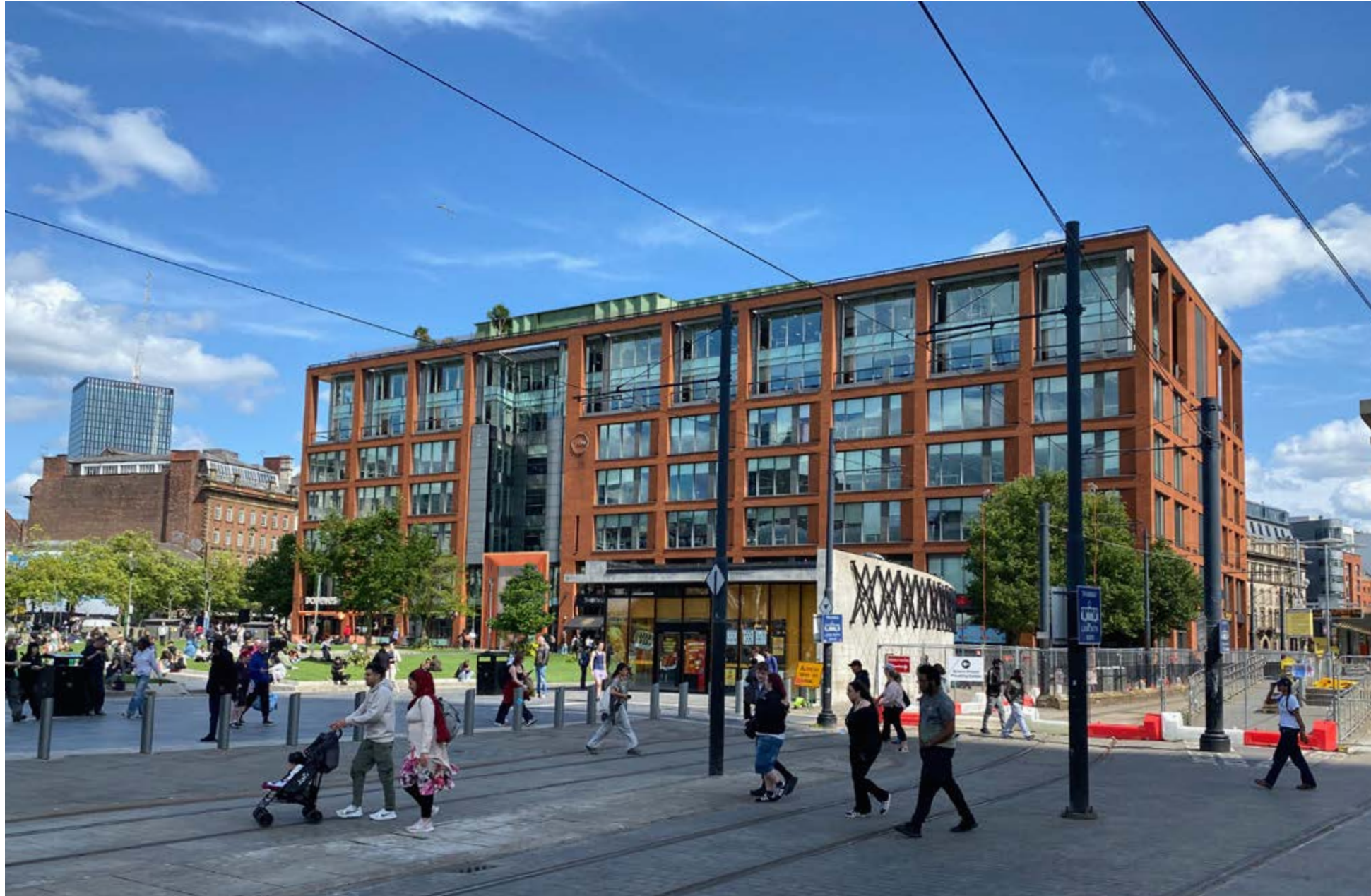
4.6 VIEW FROM MOSLEY ST.
