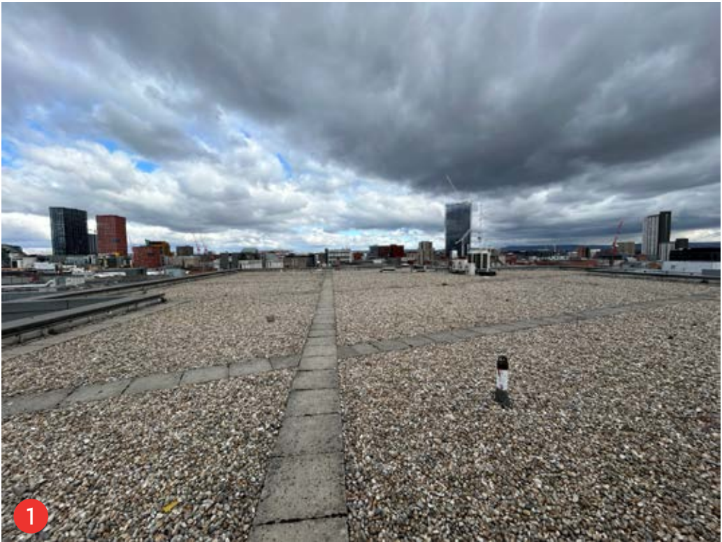
ROOFSCAPE PHOTO FACING NORTH
