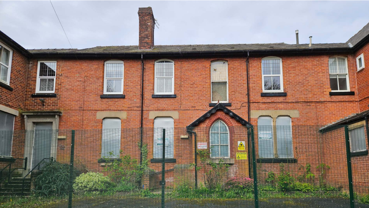
View 02 - East Elevation of St Annes House - Line of extention is visible to the left with change of brickwork and window heads/sills. Limited architectural features are present on the elevation.
