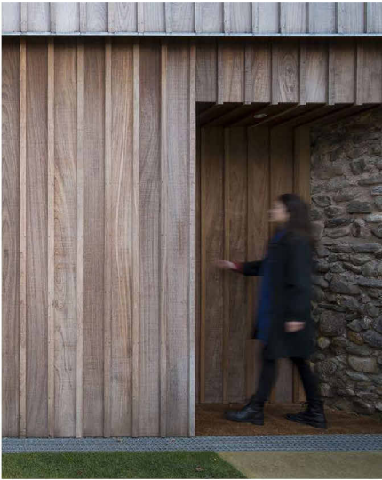
2. Vertical batten and board timber cladding
