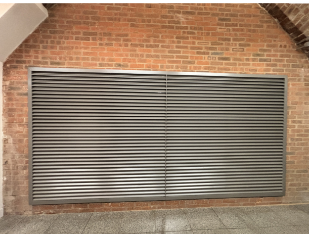
PREVIOUS NON-HISTORIC BRICKWORK INFILL WALLS TO ARCHES
