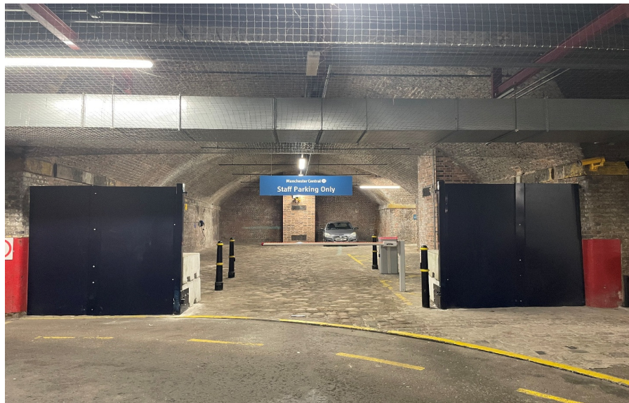
Manchester Central – VIEW 1 Basement undercroft
