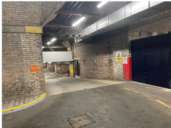
Manchester Central Convention Centre – Previously infilled arches in brickwork
