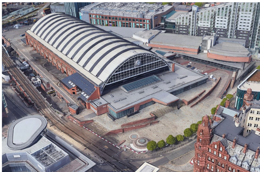
Manchester Central South-West (rear) gable view
