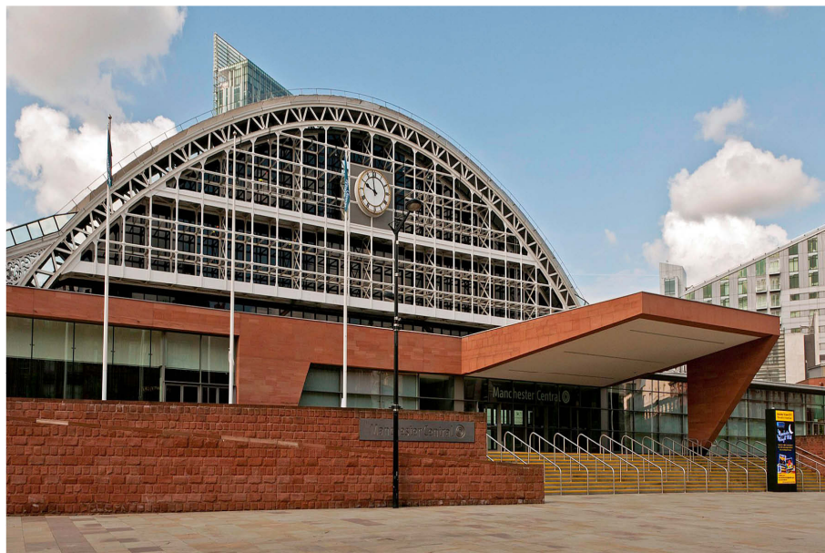
Manchester Central North-East (front) gable view
