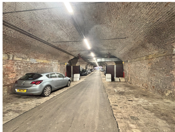
Manchester Central – View of Basement undercroft
