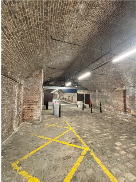
Manchester Central – View of proposed storage area
