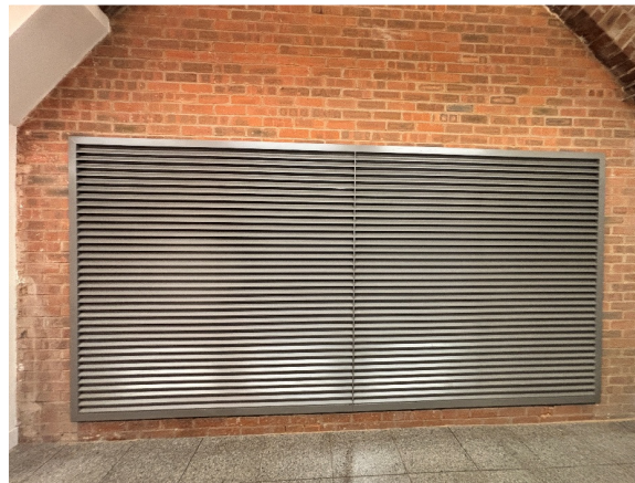
Manchester Central Convention Centre – Previously infilled arches in brickwork
