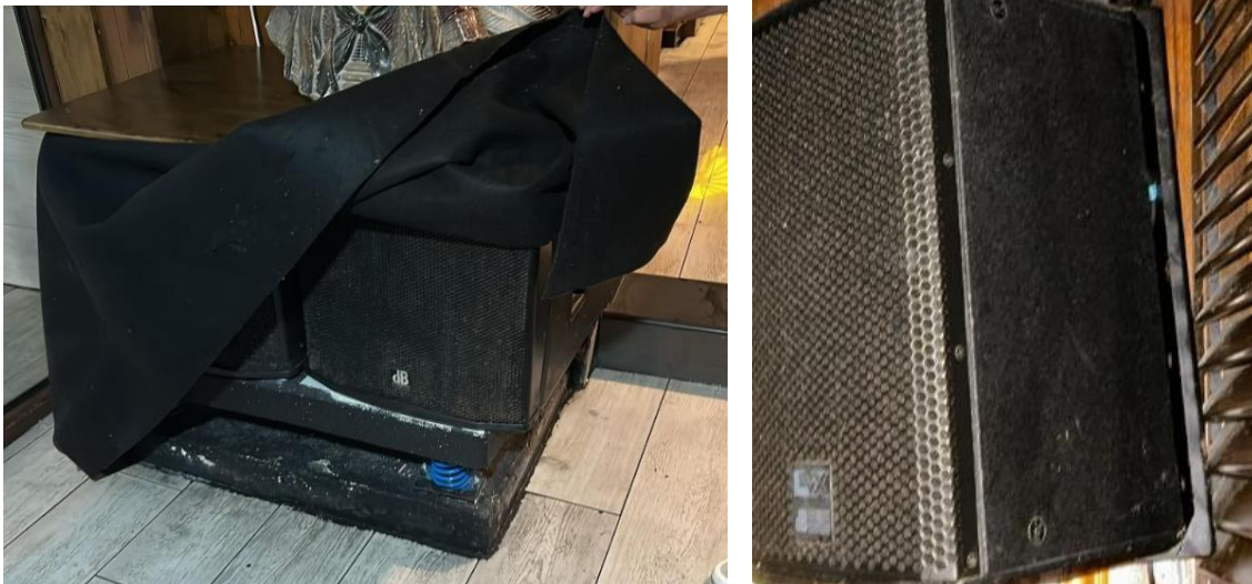
Figure 4 Example images of sound system on inertia base with steel spring mounts (left) and resilient mount (right)
