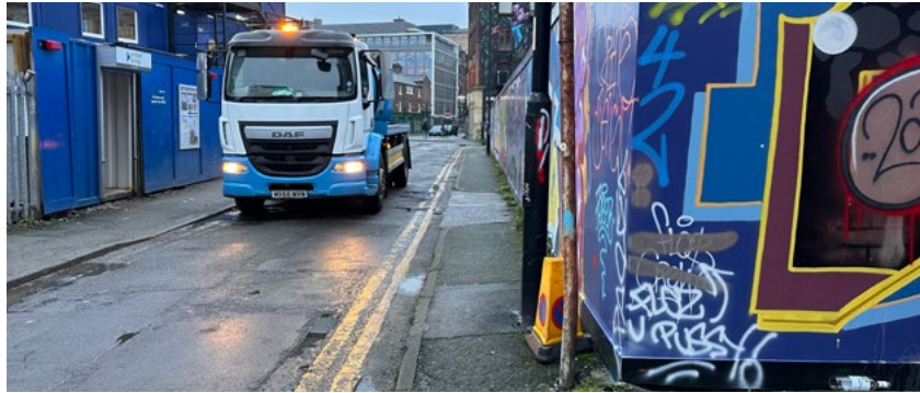
7 View from The Site on Dean Street, looking south
