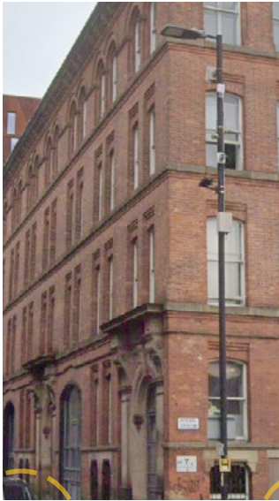
Lighting - existing columns retained T1 - Newton Street
