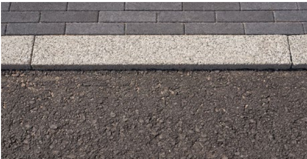
Fusion kerb edging to inside of the site & resurfaced carriageway as indicated
