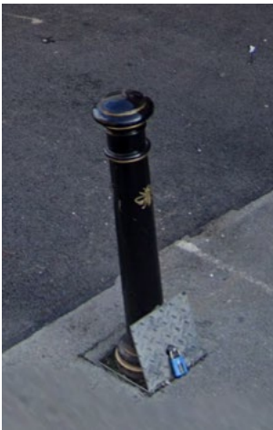
Demountable bollards, Standard MCC Spec
