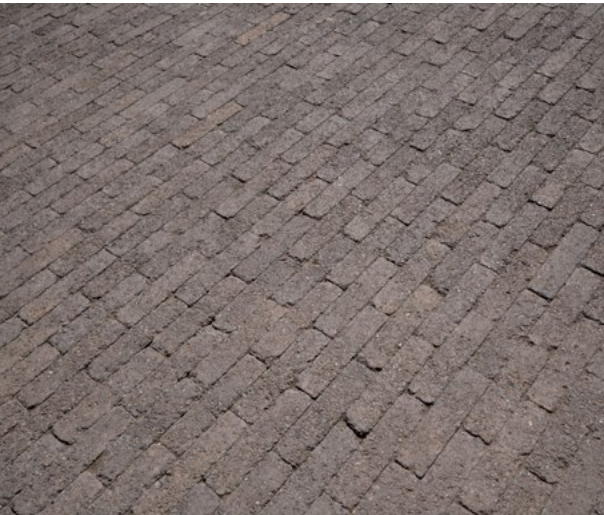
Clay style block paving New surface detailing to Newton Street. Tumbled Inish block paving: 200 x 50 x 80mm
