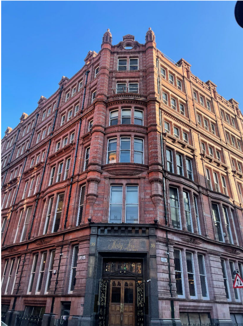
Figure 37- View of 35 Dale Street. Source: Author's own, January 2025.
