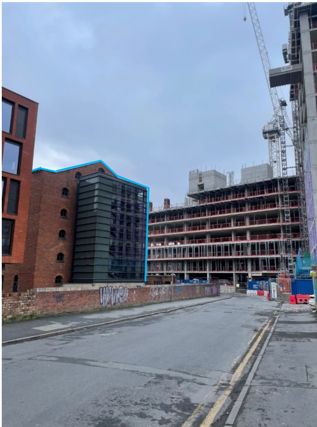
Figure 33- View of Former Rochdale Canal Warehouse outlined in blue. Source: Author's own, February 2025.
