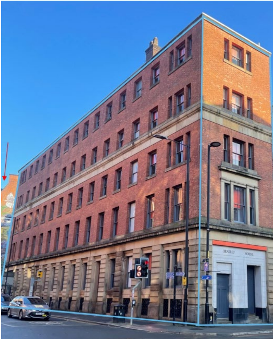
Figure 35- View of Bradley House in conjunction with the Site denoted by red arrow (approximate location and asset in blue). Source: Author's own, December 2024.
