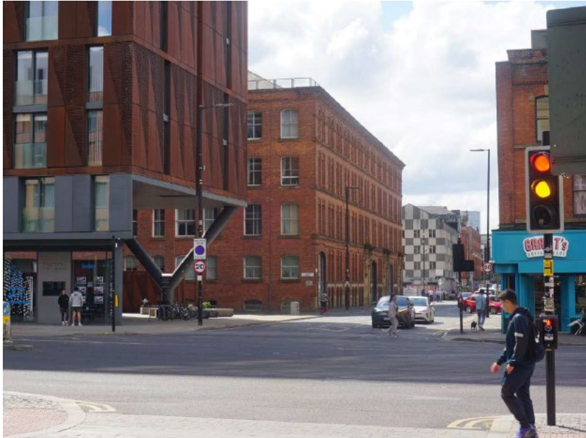
Figure 63- View 1 from Blossom Street showing 72-76 Newton Street (The Wentwood), Marlsbro House, and the Newton Buildings. Source: Re-Form, 17 December 2025.
