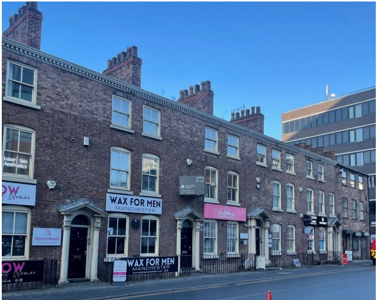
Figure 39- View of 69-77 Lever Street and 10 Bradley Street. Source: Author's own, January 2025.
