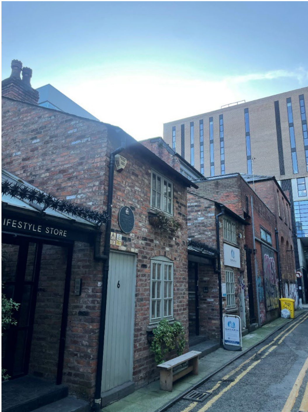
Figure 43- View of 4, 6 and 8 and attached screen walls. Source: Author's own, January 2025.
