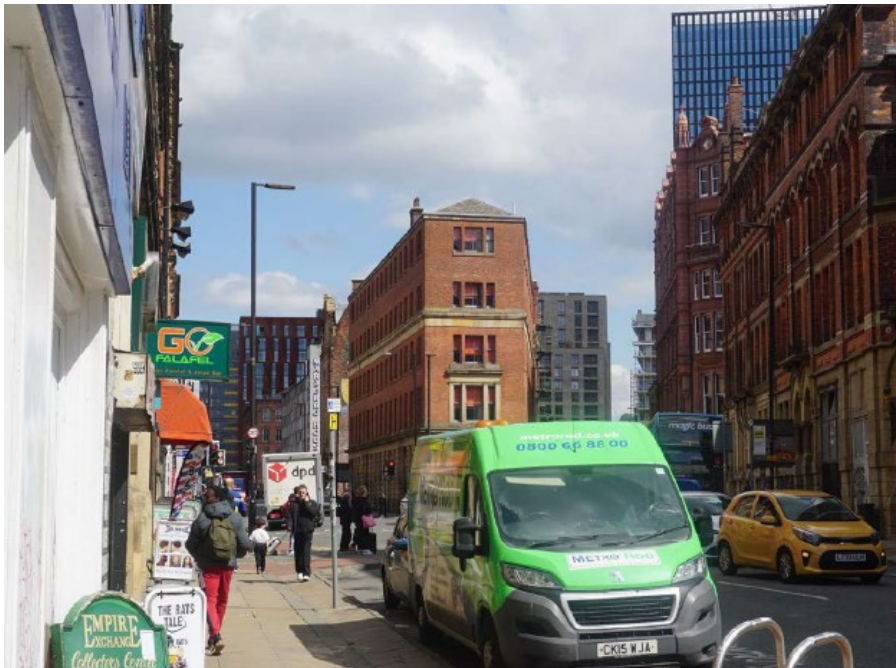
Figure 68- View 3 showing Bradley House, Newton Buildings and Marlsbro House from Newton Street. Source: Re-Form, 17 December 2025.
