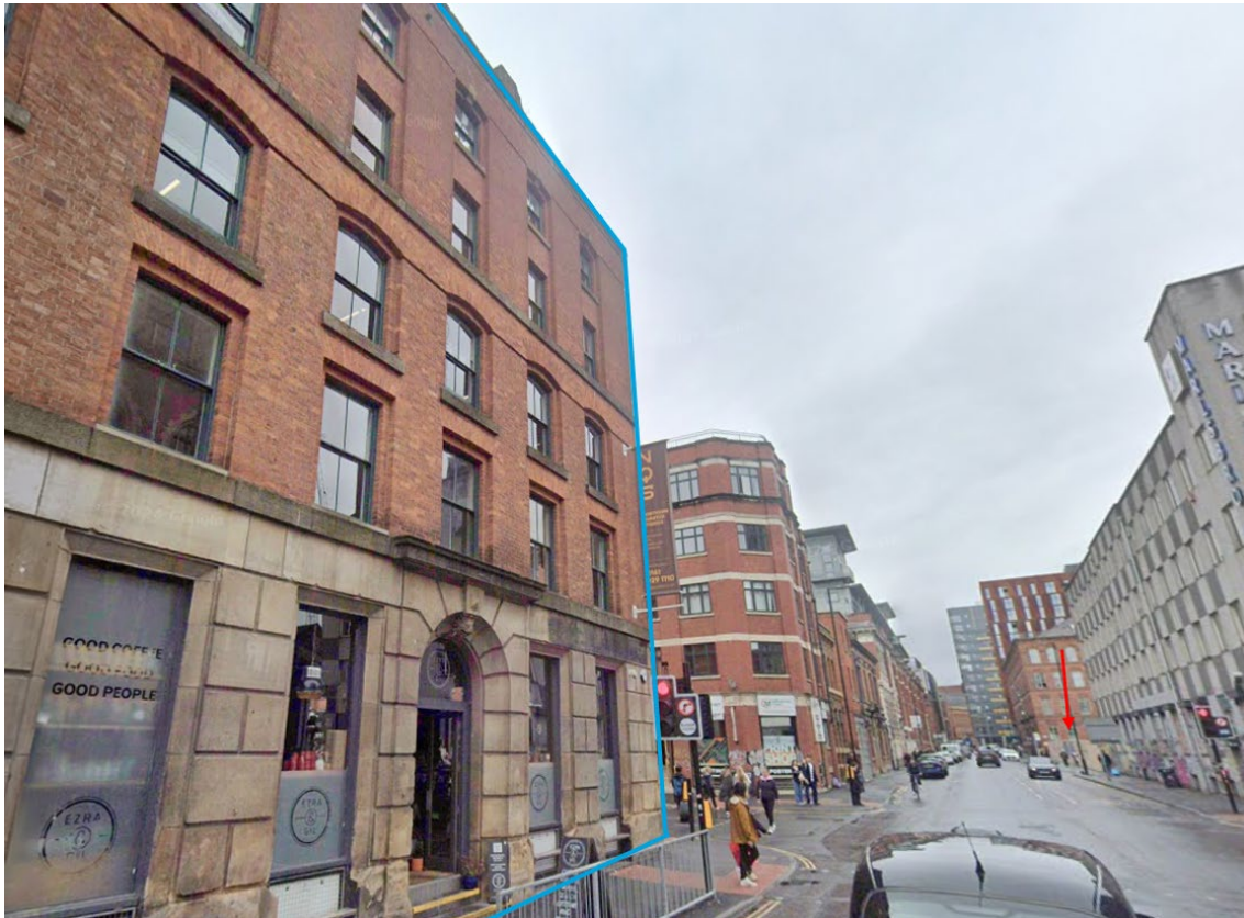
Figure 34- View of 45 and 47 Newton Street in conjunction with the Site denoted by red arrow and heritage asset edged in blue. Source: Google Maps, July 2024 (Accessed 24 March 2025).
