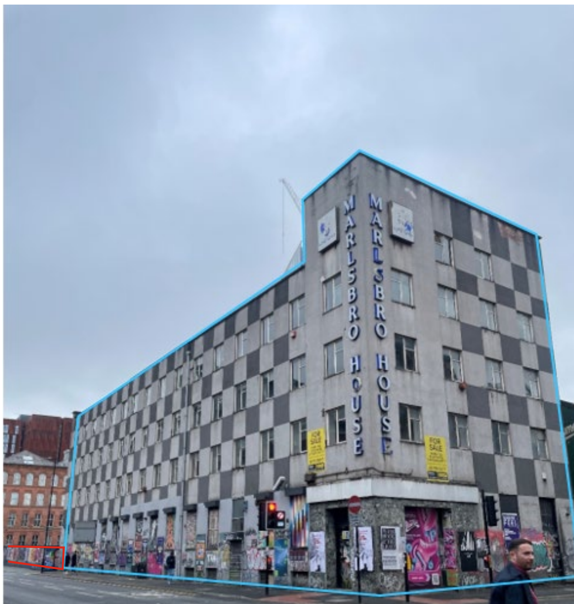
Figure 24- View of Marlsbro House in conjunction with the Site edged in red and heritage asset in blue. Source: Author's own, December 2024.
