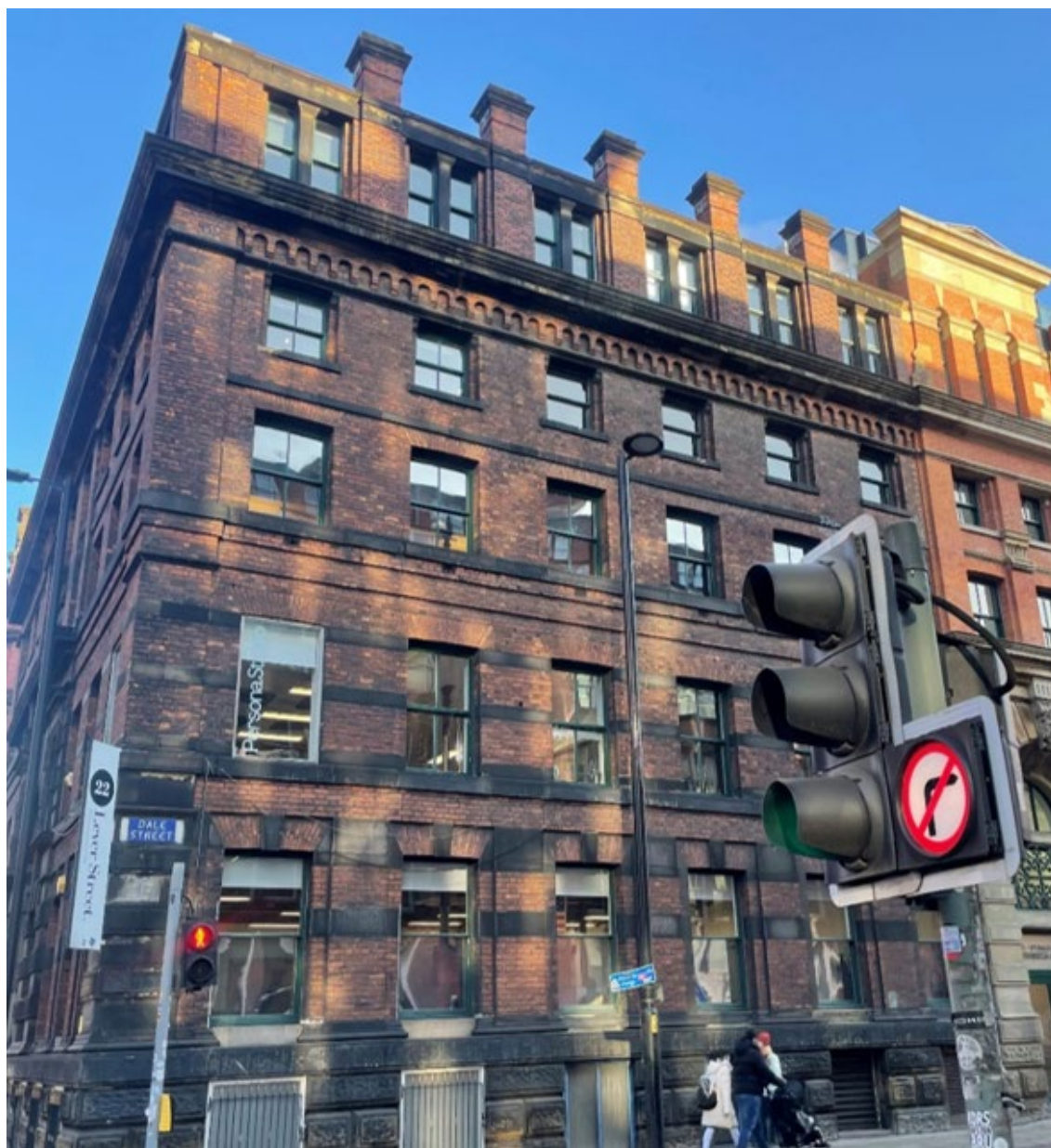
Figure 42- View of 25 and 27 Dale Street with Tribeca House in view. Source: Author's own, January 2025.
