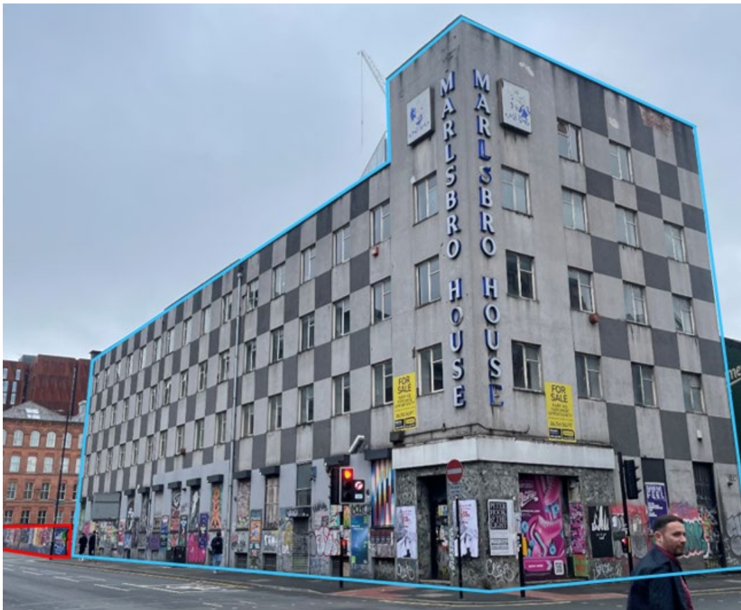
Figure 49- View of the Site from Marlsbro House. The heritage asset is outlined in blue, and the Site in red. Source: Author's own, February 2025.
