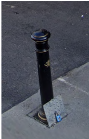
Demountable bollards, Standard MCC Spec
