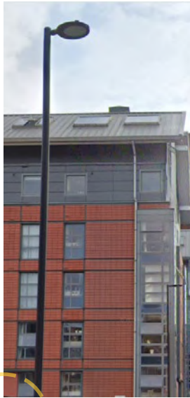
Lighting - existing columns retained T2 - Faraday and Dean Street
