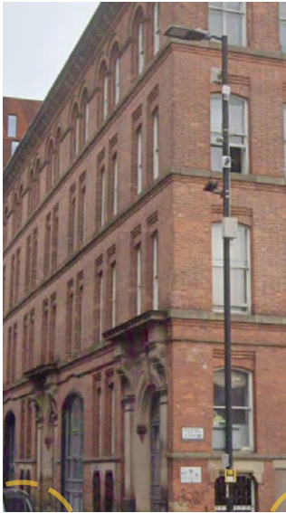
Lighting - existing columns retained T1 - Newton Street
