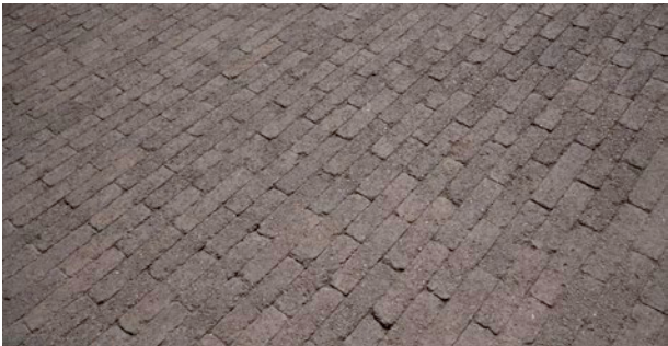
Paved entrance space Tumbled concrete block pavers, Inish by Hardscape, 200 x 50 x 80
