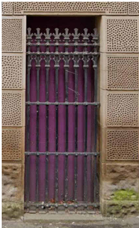
Existing Railing from Bloom St.
