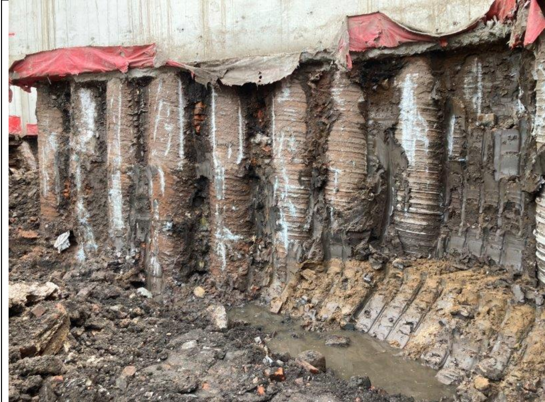
Water inundation from area of aqueduct wing wall and embankment
