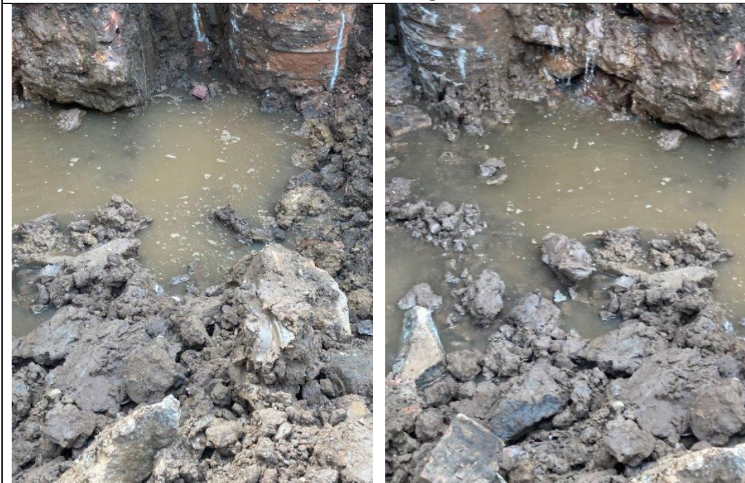
Water inundation from area of aqueduct wing wall and embankment
