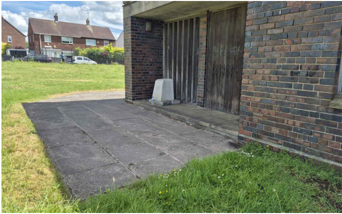
Original Main Entrance View from North-West
