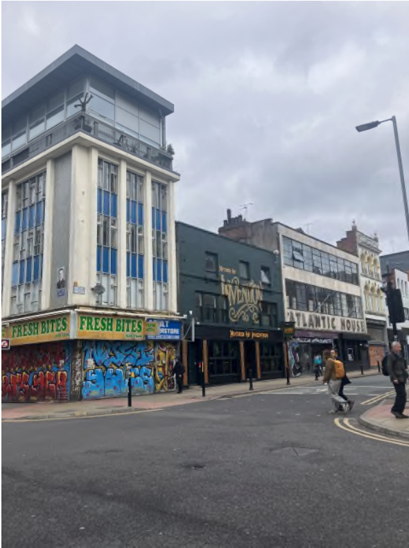
Site in the street scene
