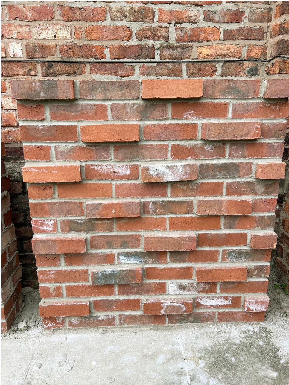
Lichfield Red Multi, Mock-up made on site, 1000mm (h) x 1000mm (w)
