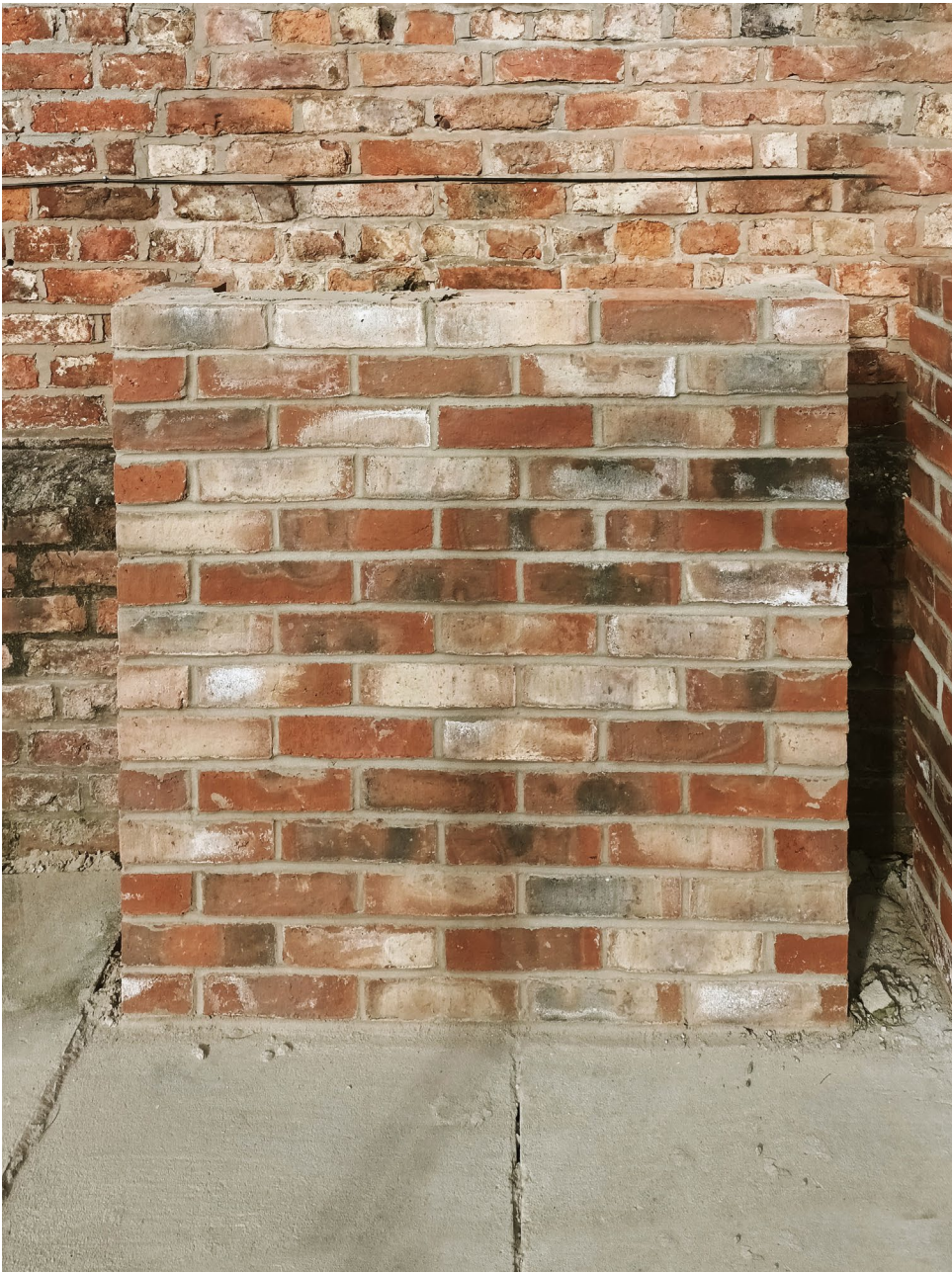
Millhouse Blend, Mock-up made on site, 1000mm (h) x 1000mm (w)
