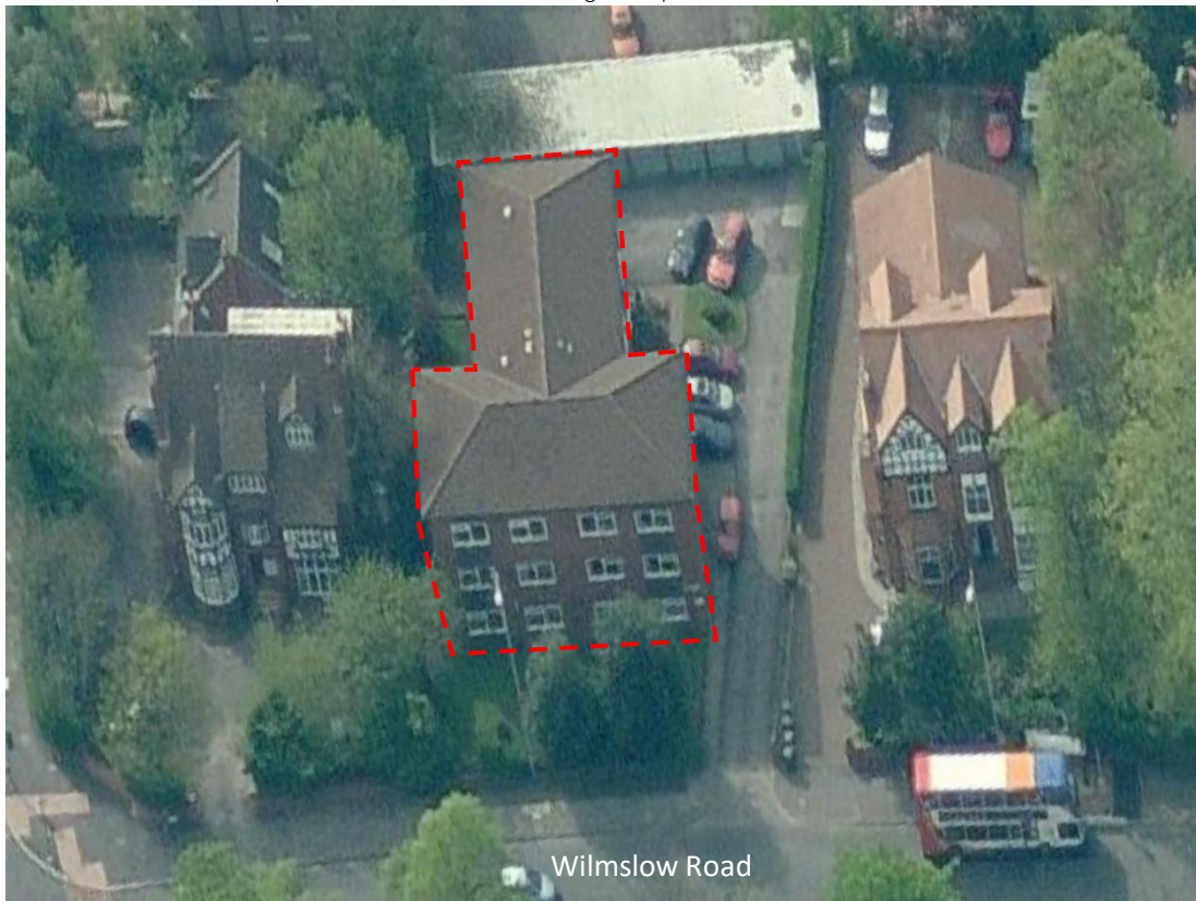
Figure 3 – Aerial view showing local context and relationship to the neighbouring buildings
