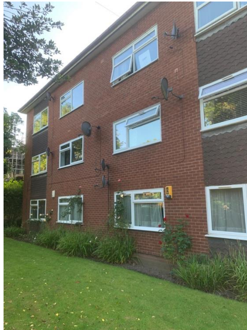
Figure 1 – East elevation of Balholm Court facing Wilmslow Road, but largely screened by well-established trees to the site boundary
